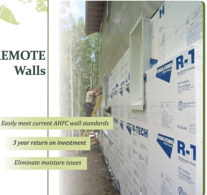
"By placing the heat, air, and moisture control layers to the exterior of the structure, the REMOTE wall system creates the perfect assembly for constructing durable, efficient, and affordable structures for all the severe climates of Alaska."
