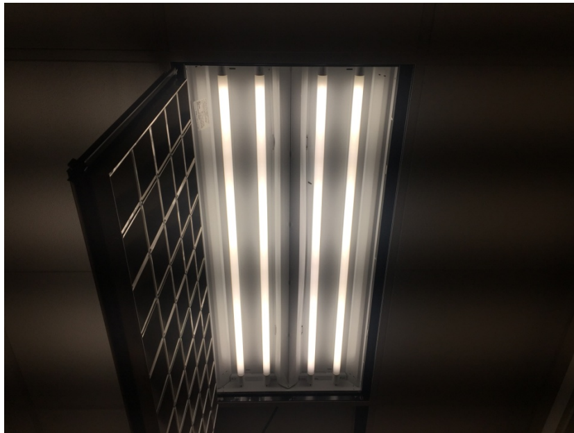
Figure 2. A cell-phone photograph may show horizontal stripes across the image from the 60Hz related flicker, as in this case, exhibited by a UL Type B lamp. Flicker modulation was not measured in this study.
