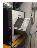
The photo to the left shows a typical HRV. In this picture, the front cover of the device has been removed, and the heat exchanger core pulled out. The core contains lots of channels – some for outgoing air, some for incoming air – and the channels allow heat to pass from one air stream to another.
