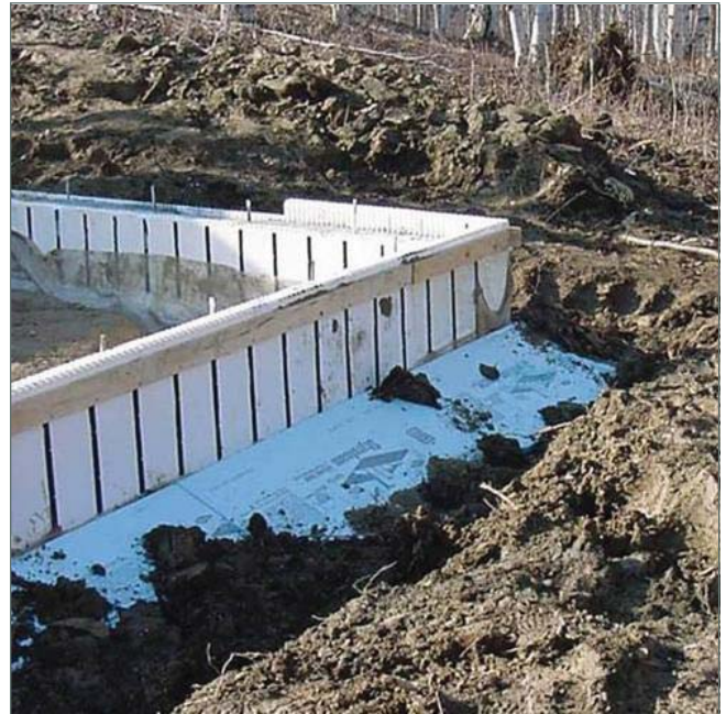
Pictured is the construction of a frost protected shallow foundation
