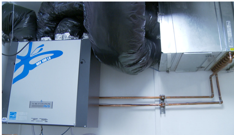
[HRV (left) and Coil Filter box (right) - Galena 2014]
