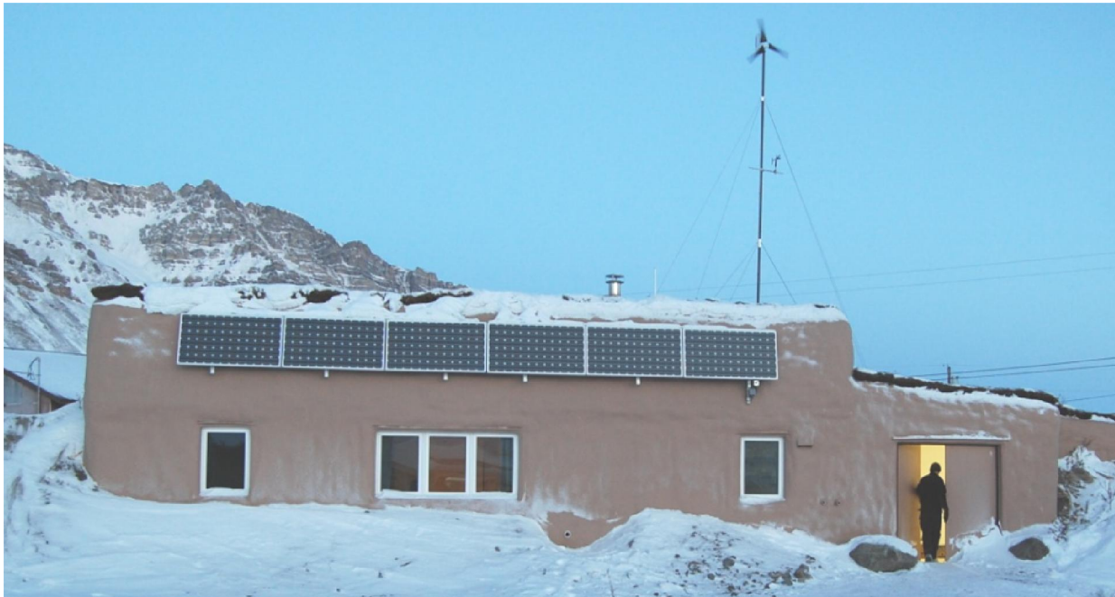
Figure 1. The Anaktuvuk Pass prototype house. The house built in 2009 has both solar and wind power generation systems installed.
