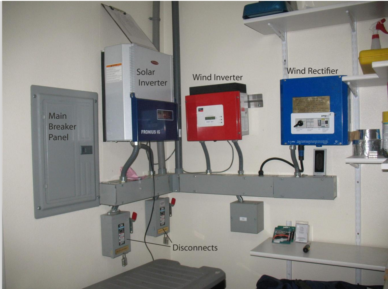
Figure 6. Interior components of the renewable energy system. These components are located in the arctic entryway, which is outside of the living space but still warmer than outside of the house.
