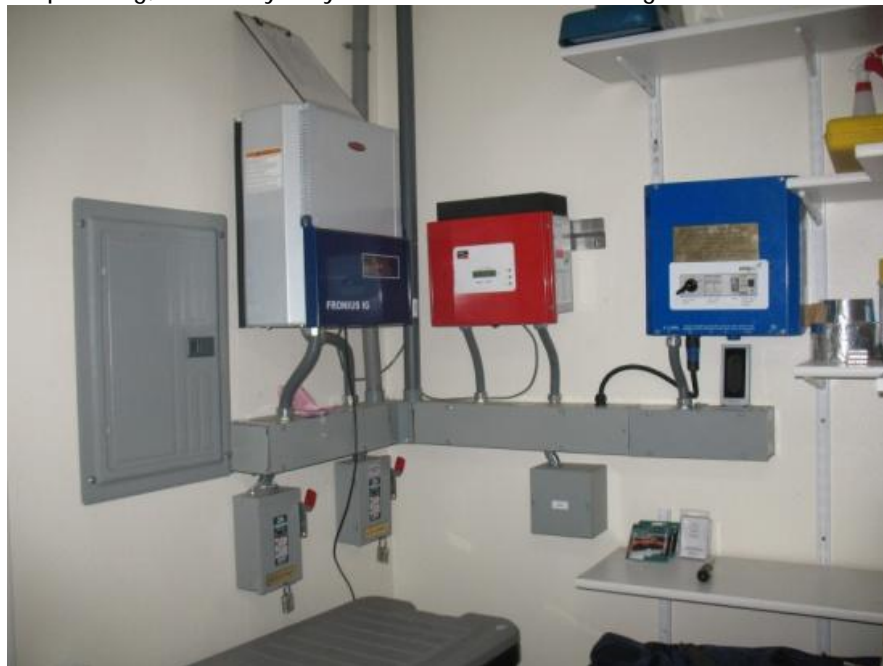
Figure 4. Inverters should be kept clean and dry.
