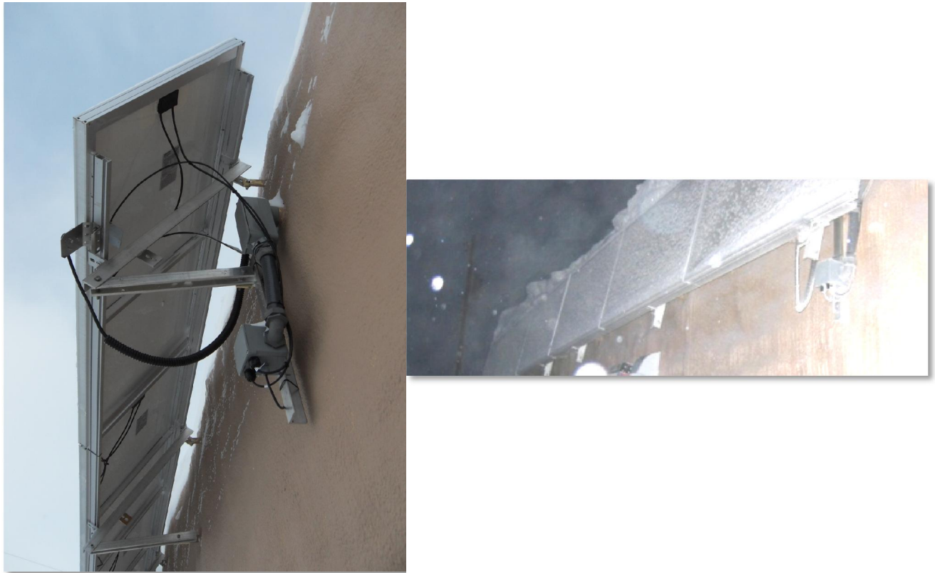
Figure 17. Solar array adjustable positions. The array can be tilted to 53 degrees from horizontal (as shown on left) to maximize solar radiation during the months without snow. The array can be tilted to 90 degrees from horizontal (as shown on right) to reduce snow cover on the panels and to maximize solar radiation during the months with snowfall.
