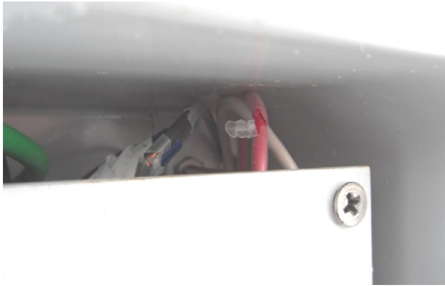
Figure 5. Cracked wiring should be replaced by an electrician.
