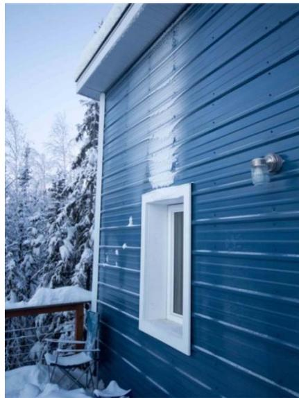
**Figure 12. Frost formation above the window was created by the vapor escaping from the open window in the Spruce house.**
