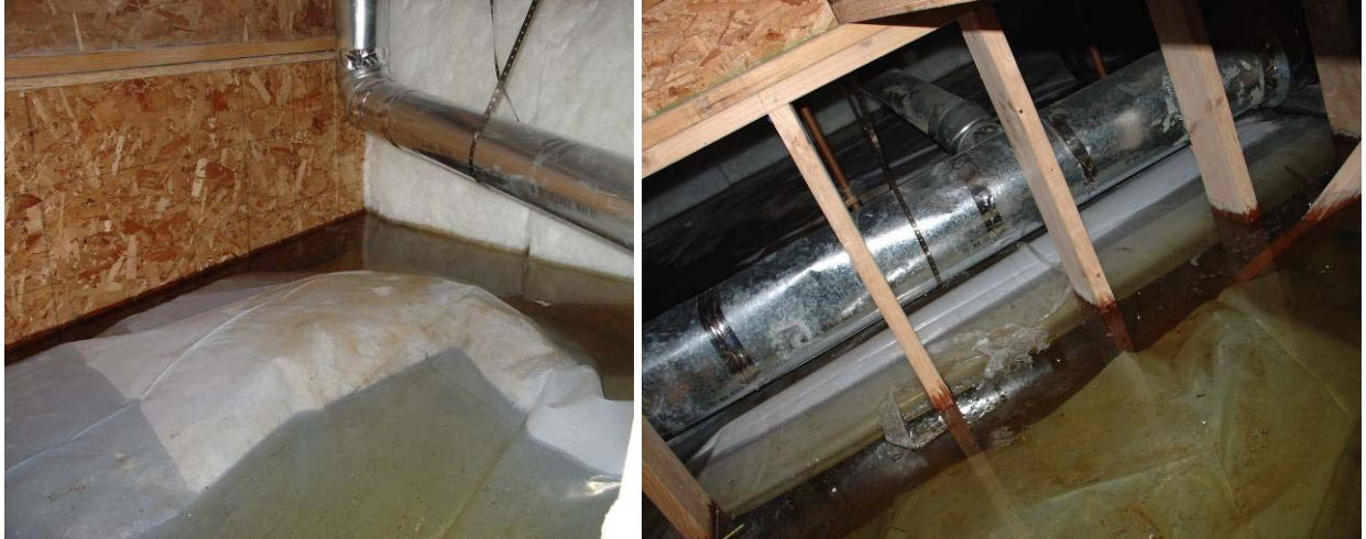
Figure 21: SC06 flooded crawl space during monitoring period.
