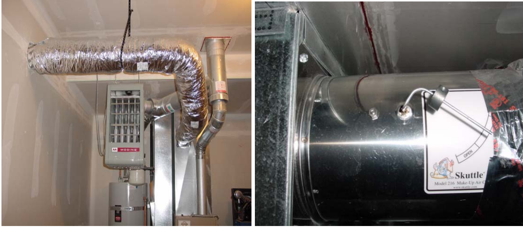
Figure 1: Outside air duct brings fresh air into the furnace return through a Skuttle damper.
