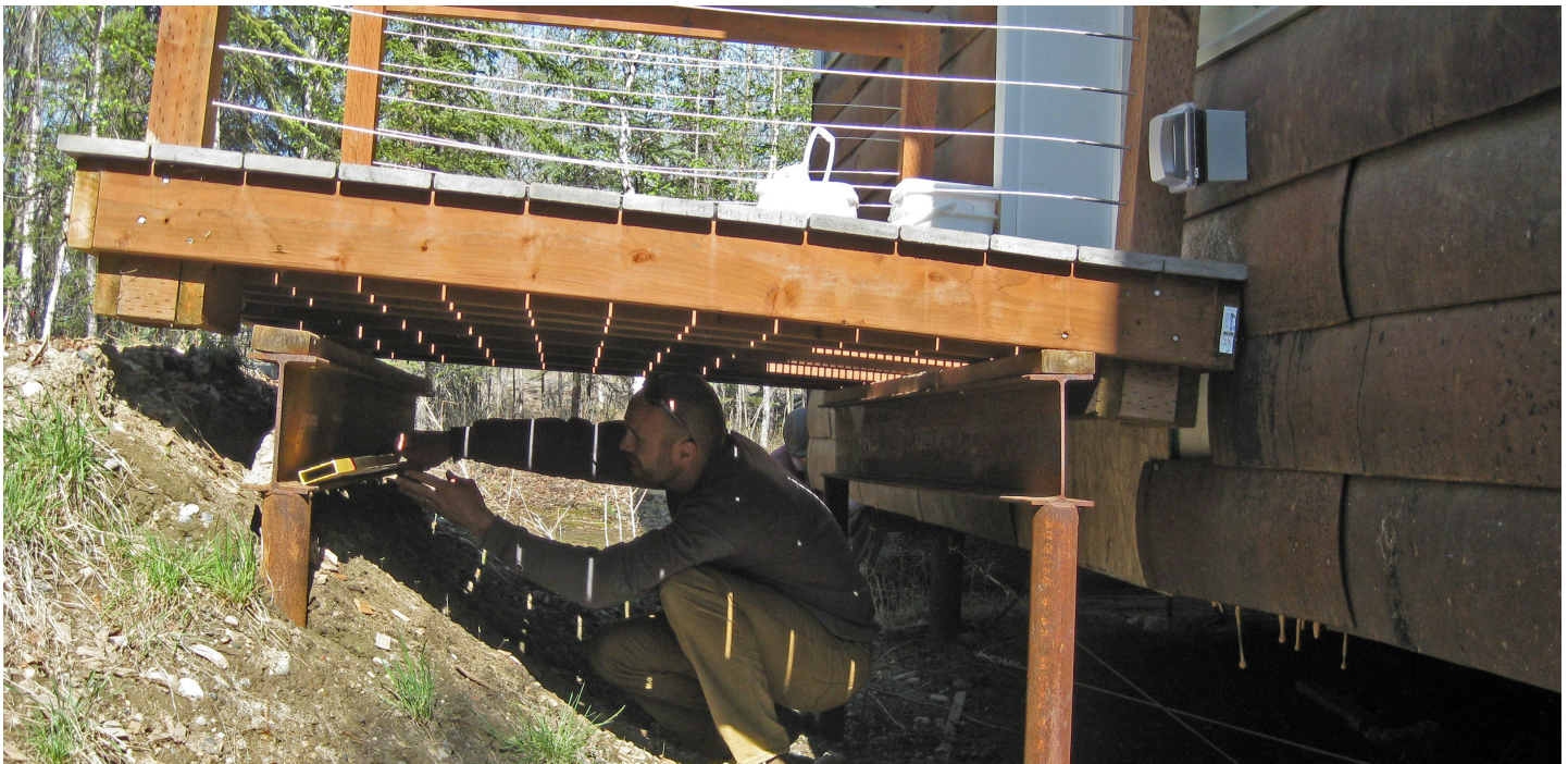
Figure 1. Frost heave of the left two pilings under the deck entry of a home in Fairbanks.
