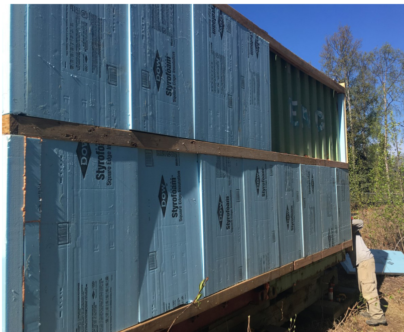
Figure 15: The AVEC storage containers received insulation to reduce their heat load and free up waste heat for use in Blackwell School.
