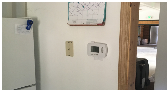
Figure 19: The weatherization crew replaced thermostats in the clinic with programmable versions to facilitate temperature setbacks to reduce energy use when the building is unoccupied.
