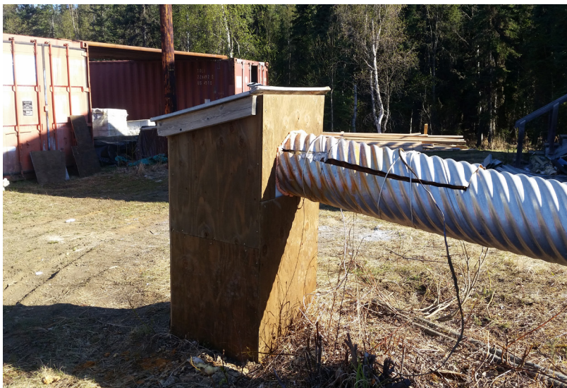
Figure 20: RurAL CAP rebuilt the well-head arctic box at the washeteria in 2017.
