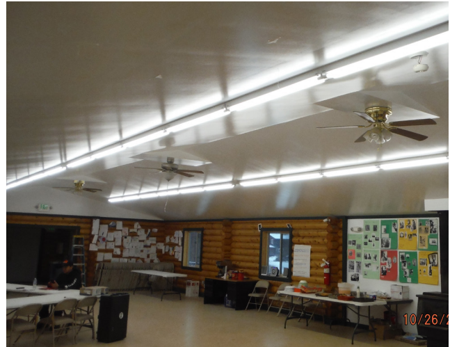
Figure 13: Installing and using programmable thermostats and a lighting upgrade were the top two energy audit recommendations for the community hall in Anvik.
