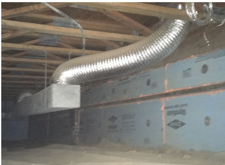
Figure 16: Crawlspace retrofits included insulating the walls and adding a vapor barrier to the floor.
