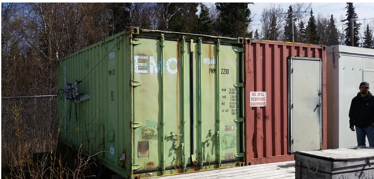
Figure 2: The storage containers for the power plant did not have insulation prior to the SPARC retrofit project, and used the vast majority of the heat available from the heat recovery system.
