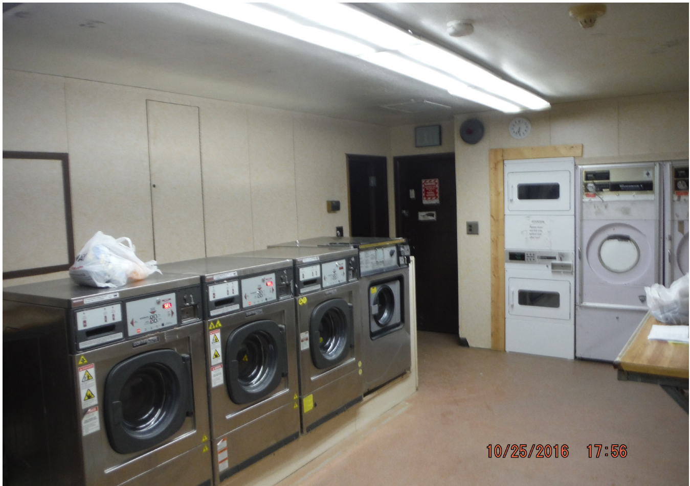
Figure 14: The top audit recommendation for the Anvik washeteria is to replace the electric dryers with hydronic versions.
