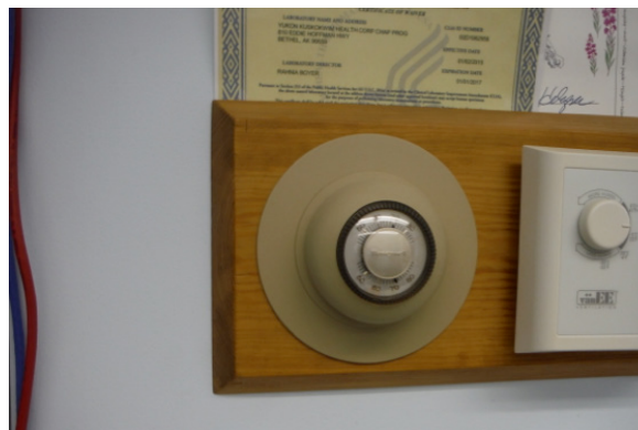
Figure 12: The top audit recommendation for the clinic is to replace existing thermostats with programmable versions.
