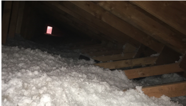
Figure 17: A crew air-sealed and insulated the city office building attic.
