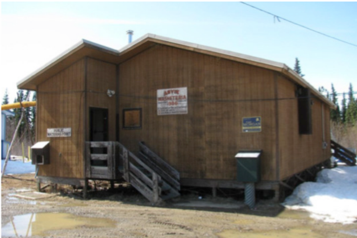
Figure 10: The water treatment plant and washeteria building contains water distribution, a laundromat, and showers for community members.
