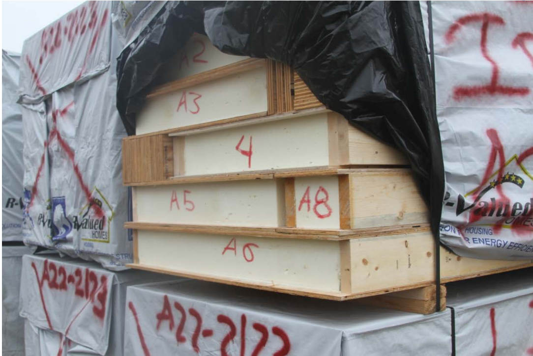
Figure 3: Panels should be protected from moisture when stored on a job site.
