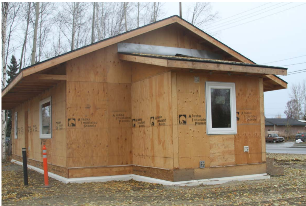
Figure 12: An IRHA house being building with SIPs in Fairbanks.
