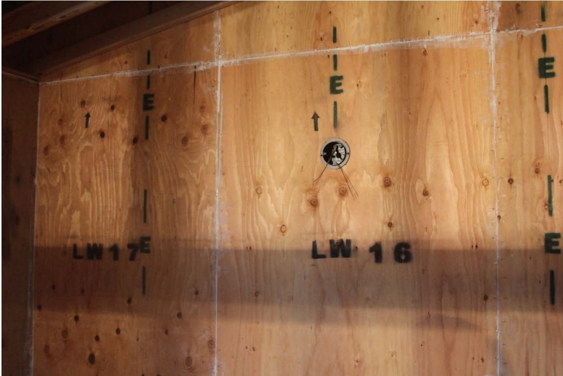
Figure 7: Panels must be sealed together where they join.
