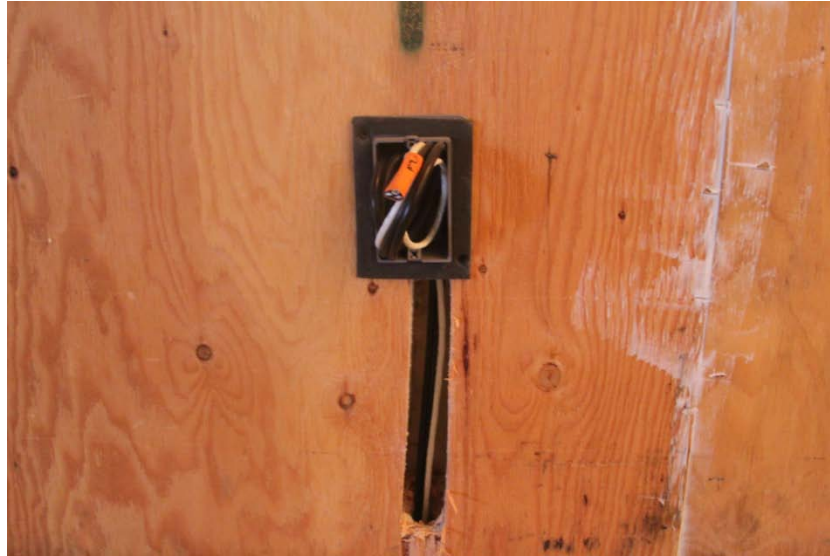
Figure 4: Channels for electrical fixtures are pre-cut in the panels at the factory.
