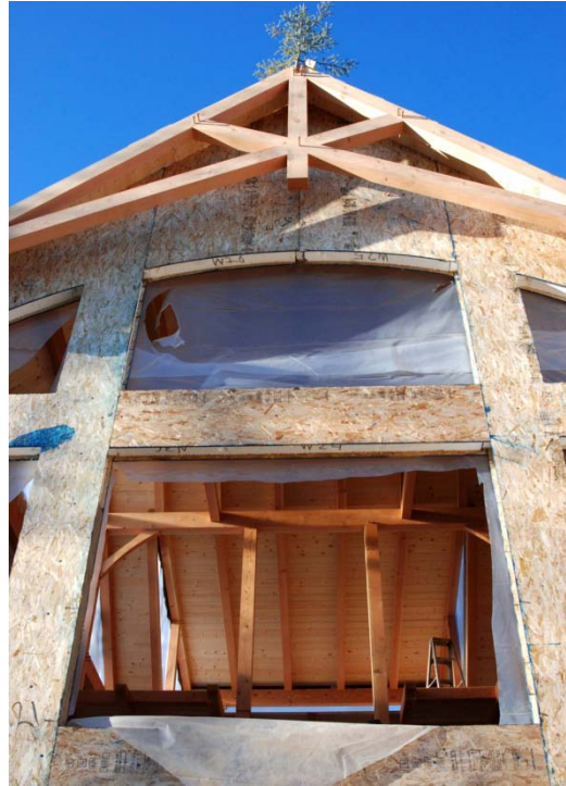
Figure 5: A house with SIP walls ready for finishing. Photo courtesy Dave Miller of Landmark, Inc.
