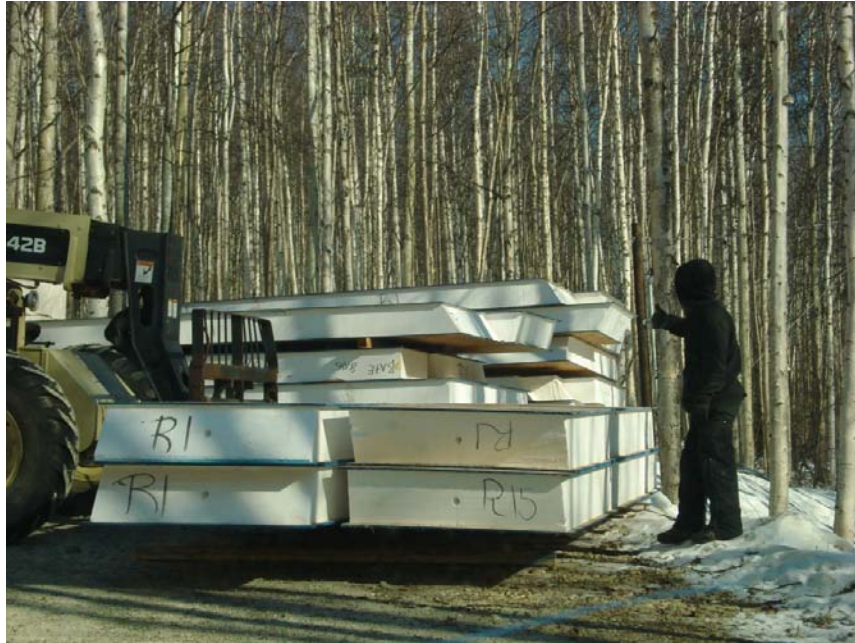
Figure 1: SIPs are numbered at the factory so that builders know where to place each panel. Photo courtesy Dave Miller of Landmark, Inc.
