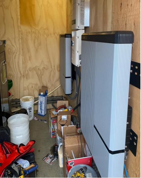
Figure 3: The inverter and two batteries for the Tribal Office solar PV system. The batteries store electricity produced during the day to be used at times when their is no sunshine, increasing the amount of solar electricity used by the building.
