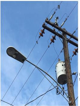
Figure 1: The streetlights in Ruby were converted from high-pressure sodium to LED lamps in Fall 2017.
