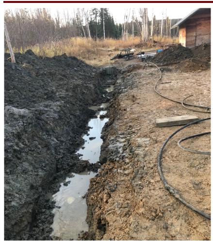
Figure 5, left: The header ditch for the ground source heat pump ground loop near the Tribal Office.
