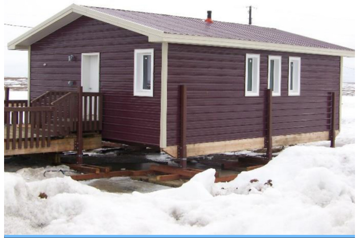
The new design has a post-on-pad foundation that isolates the heated building envelope from the frozen ground.
