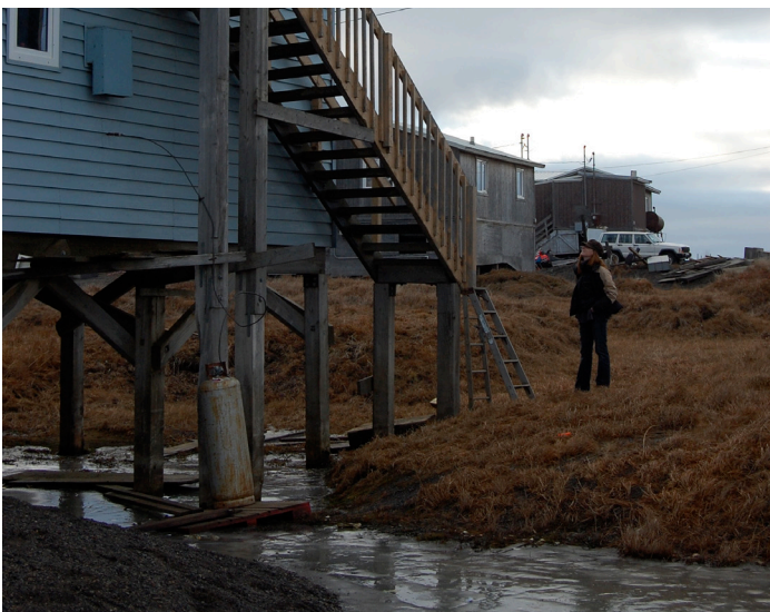
Water pools under a house in Point Lay, as wood pilings conduct heat to the ground during the summer and thaw frozen soil. This process can cause subsidence of up to 5 feet for homes on the North Slope.
