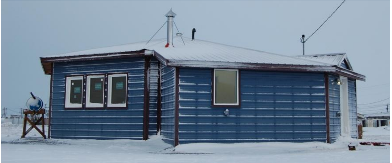
Figure 1. Quinhagak prototype house after a wind driven snow storm. The shape of the house sheds the wind and does not create large drifts in areas that would block the doors or windows.
