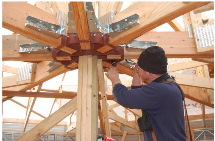
Figure 9. The roof system. The trusses were small enough that the six person crew was able to raise them without heavy machinery.
