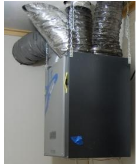
Figure 3. Quinhagak prototype house ventilation system. This high efficiency HRV is located in the mechanical room and circulates fresh air throughout the house.
