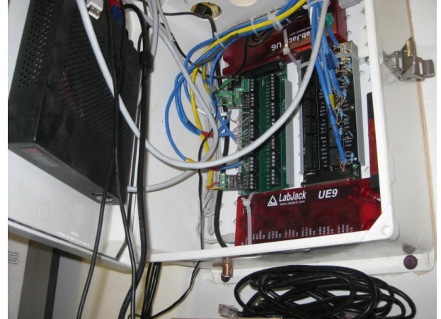
Figure 4. Quinhagak Datalogging System. The datalogging system fits in a small box in the mechanical room.
