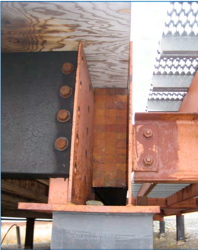
Above: The decking overhangs the long side of the structure, protecting the Glulam beam. On the short side, it ends flush.
