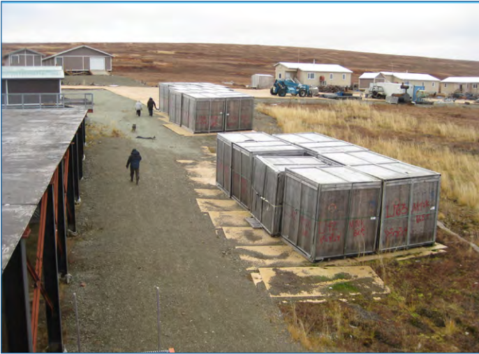
Above: The crated SIP panels are staged on Durabase mats adjacent to the existing MEC foundation.
