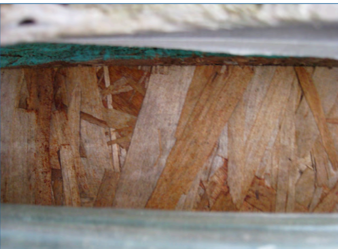
Above: the SIPs still within their protective crating appear to be as yet undamaged by the elements and should still be usable.
