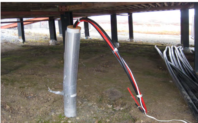
Above: A well and septic have already been installed adjacent to the MEC foundation.
