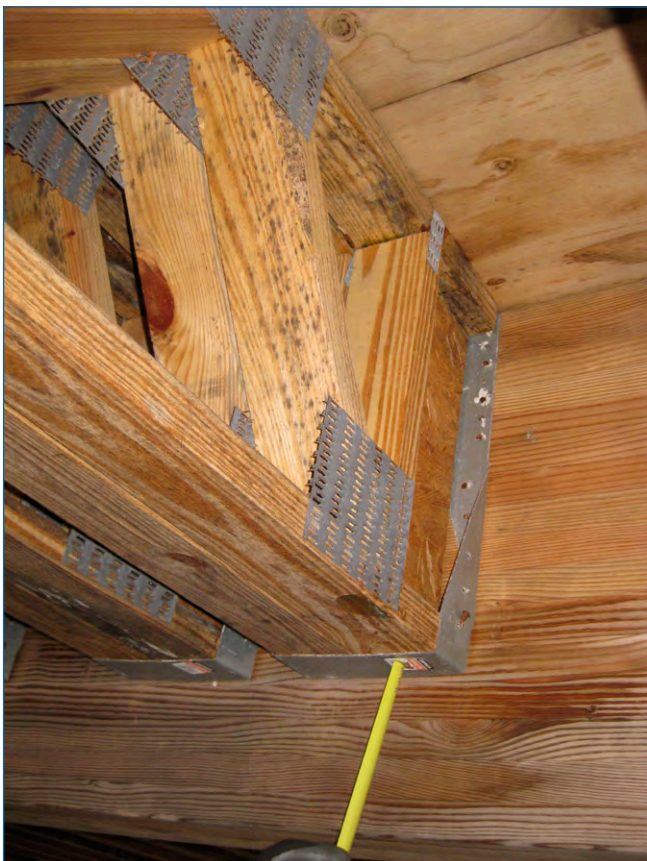
Above: Water has begun to infiltrate the temporary decking above the structure. Water can be seen wetting structural members from above.
