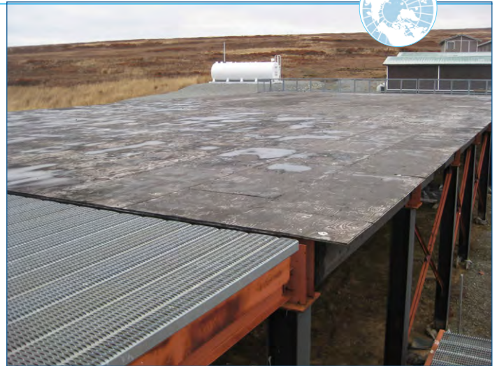
Above: The sacrificial decking meant to protect the floor is beginning to degrade and let water down in to the structural members
