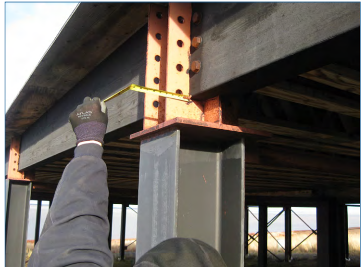
Above: The perimeter Glulam beams and steel columns appear to be in good condition.
