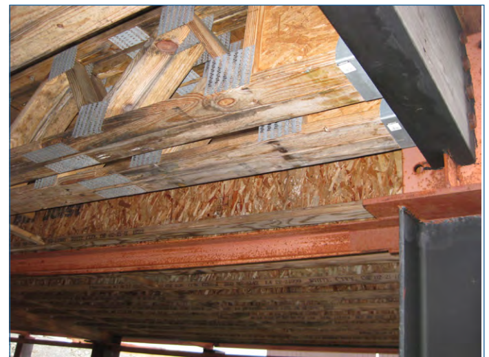
Above: Discoloration of structural joist members by water infiltration through the decking.
