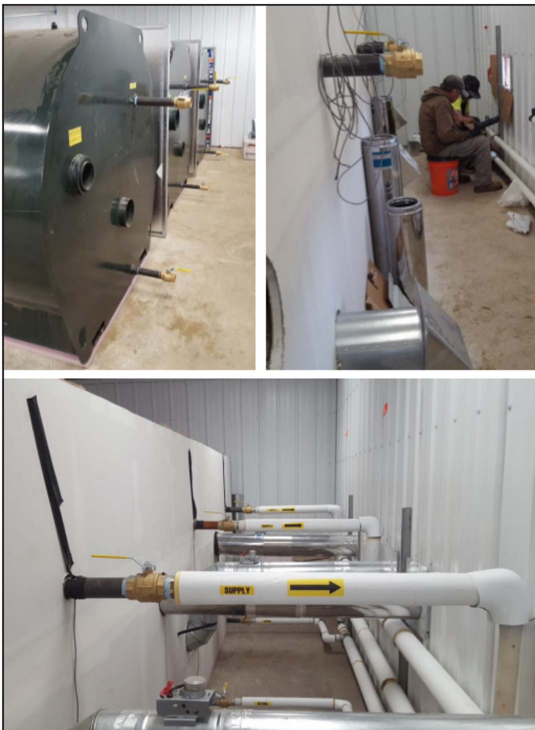
Figure 5: Top left: backs of boilers before any connections were made. Top right: back of the boiler enclosure, showing the glycol pipes, exhaust pipe, and hole for inlet air (awaiting a connection). Bottom: all connections to the back of the boilers, completed and labeled. Photos courtesy of Dave Pelunis-Messier.
