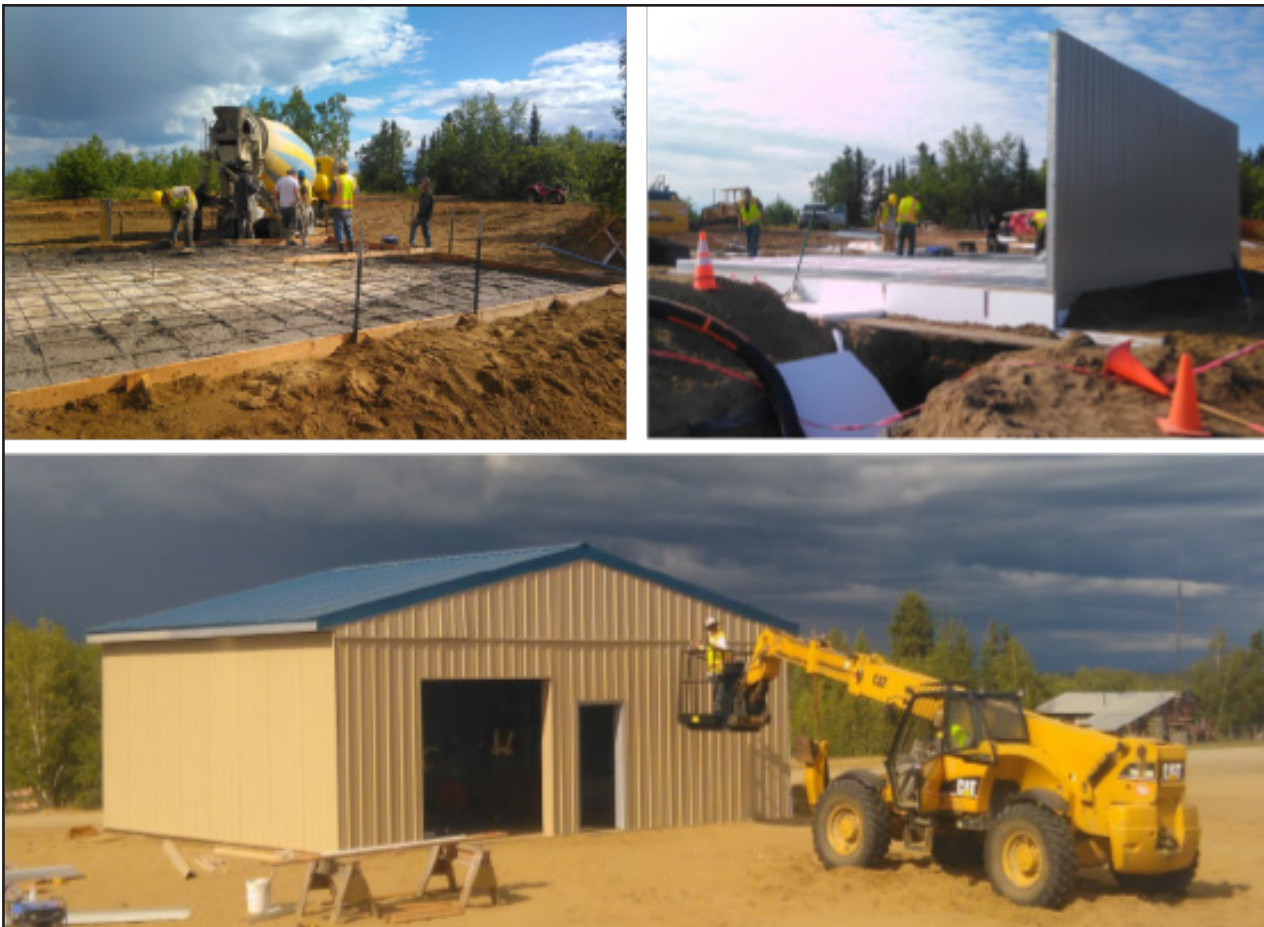
Figure 3: Construction of the biomass building. Top left: pouring of the concrete foundation. Top right: raising of the walls plus the trench for the glycol run. Bottom: nearly completed biomass building. Photos courtesy of Dave Pelunis-Messier.
