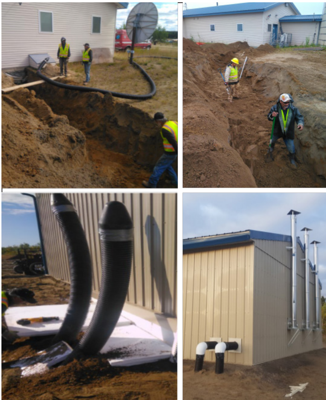
Figure 6: Distribution system includes Ecoflex thermal twin pipes carrying the heated glycol underground from the biomass building to the other buildings. Top row, left to right: trench by clinic is ready for the insulated pipe; trench to the water treatment plant is being backfilled. Bottom row, left to right: the pipes come up adjacent to the biomass building prior to connection; once complete, the connections go through the wall, leaving two elbows visible next to the building. Photos courtesy of Dave Pelunis-Messier.
