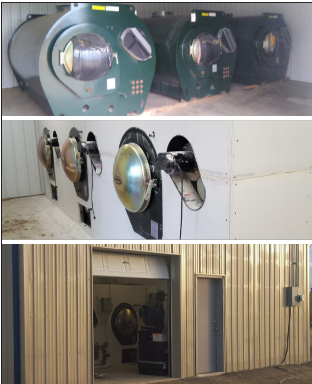
Figure 4: Top: Biomass boilers waiting for installation. Middle: Boilers being enclosed. Bottom: Installed biomass boilers visible through the open garage door. Photos courtesy of Dave Pelunis-Messier.
