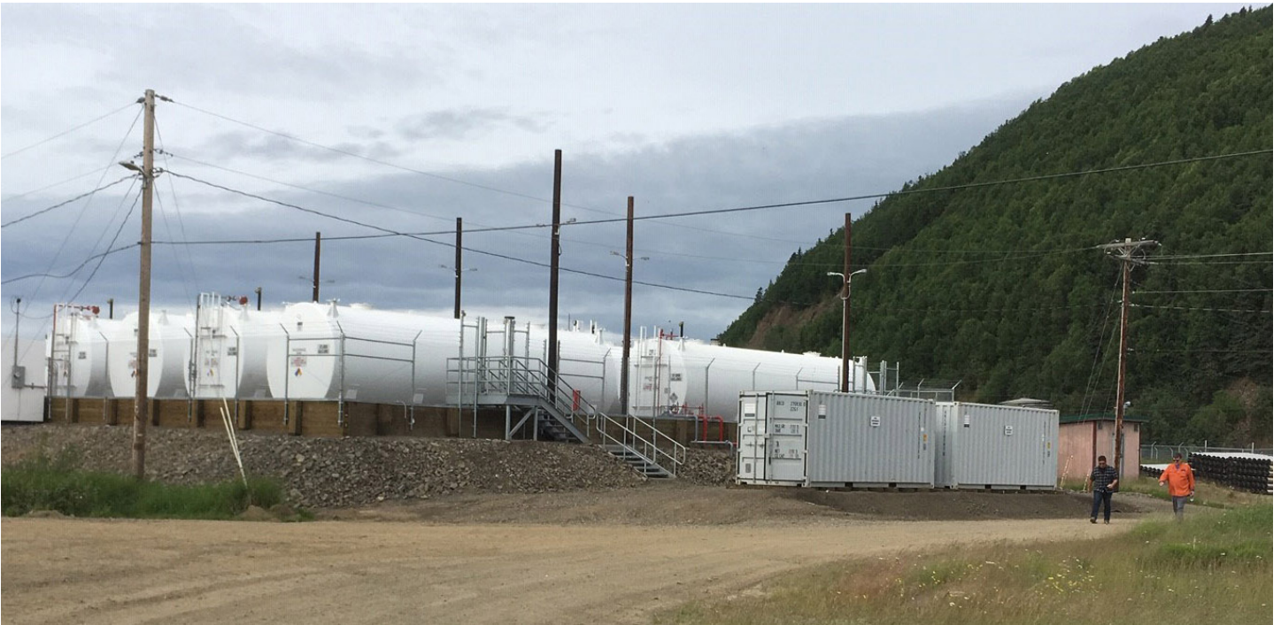
Figure 6: The tank farm serving the power plant and buildings in Holy Cross. A waste heat recovery system was added to the power plant to reduce fuel use. Photo courtesy of AVEC, 2019.
