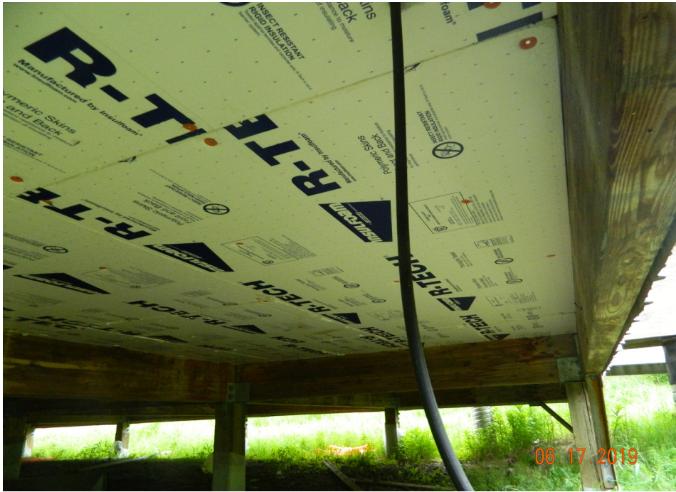
Figures 2 and 3: Weatherization improvements in Holy Cross buildings included exterior insulation under floors (above) and on walls (below).
