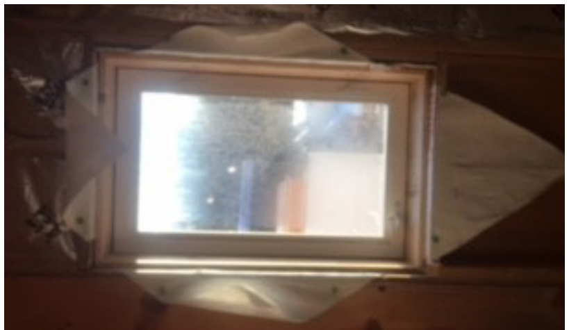
Figure 1: Weatherization improvements in Holy Cross buildings included new windows.
