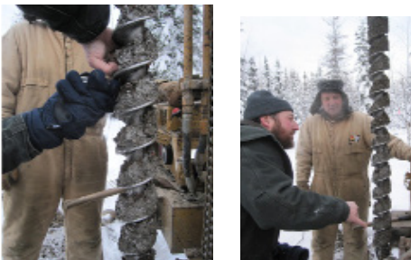
A drill rig bringing up a soil sample
