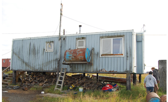
Durable housing is critical in a climate like southwest Alaska, where homes face driving rain and snow throughout the year. This home in Quinhagak has been so compromised by moisture that it is structurally unsound.
