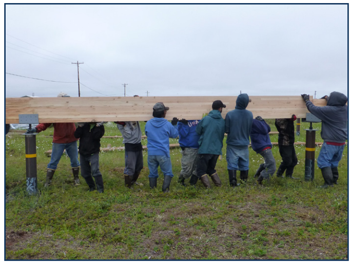
Fig 2.2 All hands on board, the beams are lifted beams into place. The center midpoint of the beams should be aligned with the previously marked spot on the center foundation supports.
