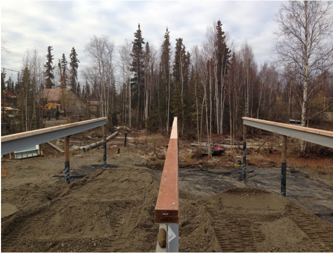
Fig 2.9 Plates can be centered over the flanges of the beams. Areas that will be covered by decks and exposed to the weather will require treated wood plates.
