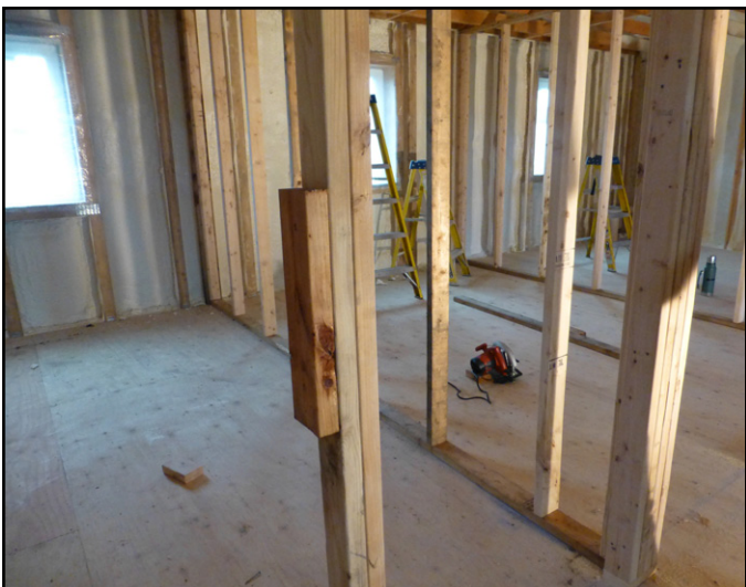
Fig 7.12 Blocking for light switch.
