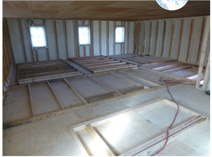
Fig 7.9 Once the ceiling is installed, the interior partitions may be framed and tipped up.
