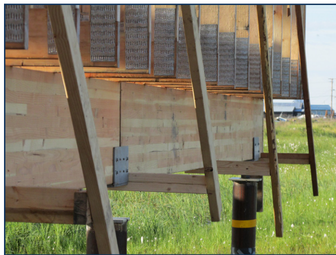
Fig 3.15 There are many methods to brace the trusses, depending on the type of foundation and beam support. It is important to have the trusses properly braced to maintain a safe work site.
