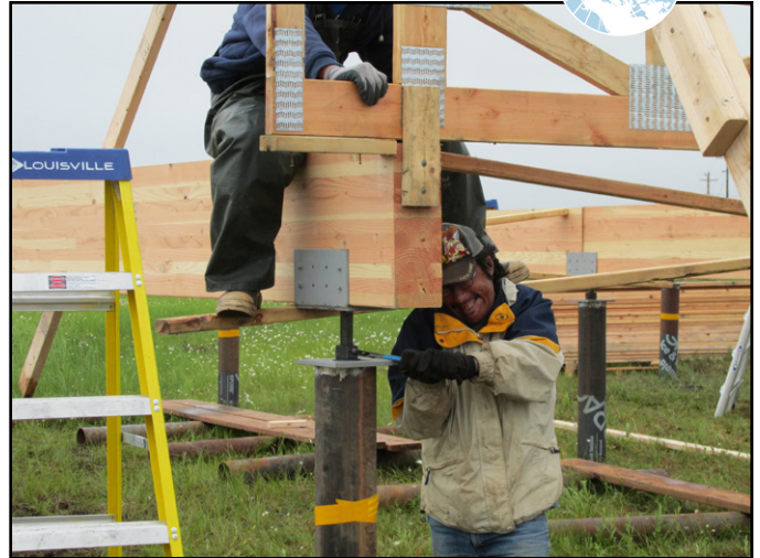
Fig 2.4 In this particular adjustable foundation design, the brackets are fastened to the glu-lam beam using carriage bolts or structural log screws, and the structure is brought to level using a wrench. In non-adjustable foundations, this will not be necessary.
