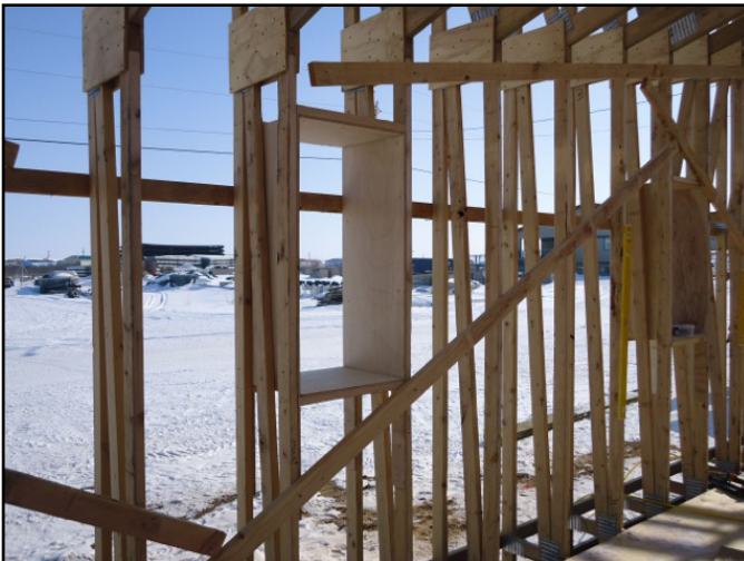
Figure 0.7 A modified version of the Integrated Truss with eave window placement between trusses in the Northwest Arctic Village of Buckland
