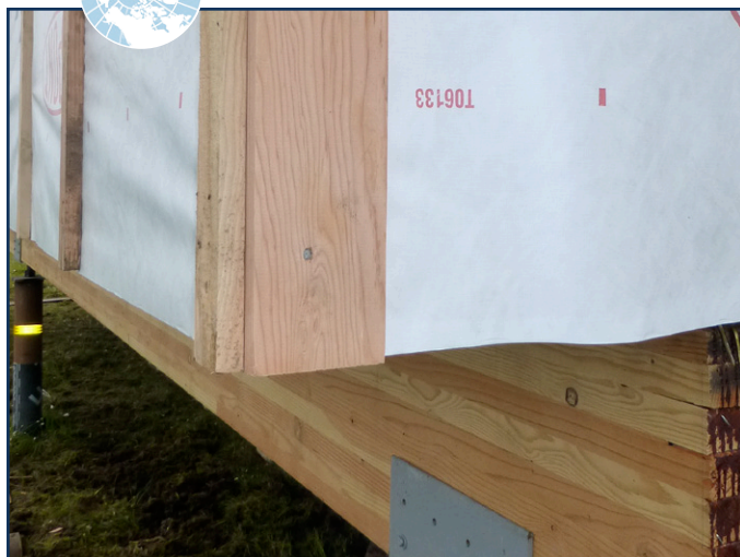
Fig 4.9 Outside corner of spacers attached.
