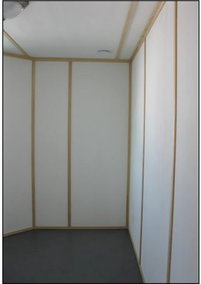
Fig 9.2 Batten strips have been stained and placed after all other finish work is complete.
