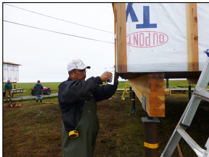
Fig 4.10 Installing insect screen at bottom edge of the building, allows air movement, prevents insect infiltration.
