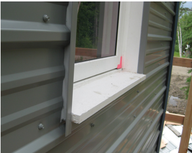
Fig 5.5 Site built exterior window jamb extension. Note the sill extends proud of the wall by up to an inch.
