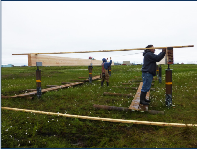
Fig 2.3 Squaring the foundation. Do not assume that the driven piles are square.
