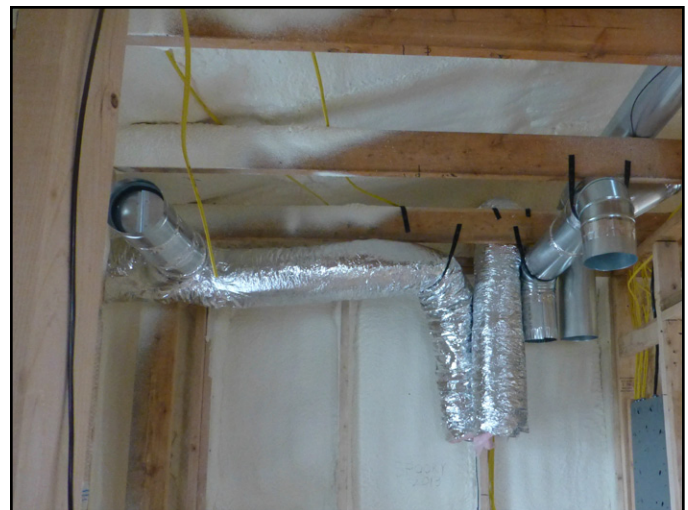
Fig 8.3 Mechanical ducting should be installed after the spray foam insulation and before the ceiling. Ducting to the outside must be insulated to avoid condensing. Warm-side supply and return ducting can be uninsulated. Refer to the installation manual of the HRV for port configuration.
