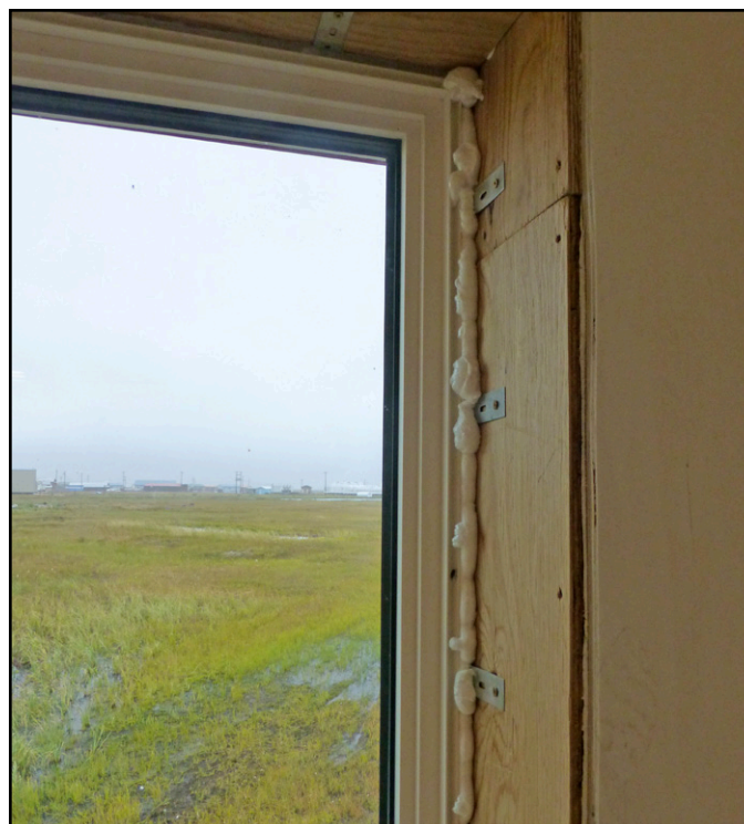
Fig 7.17 Foam air sealing around window rough opening.
