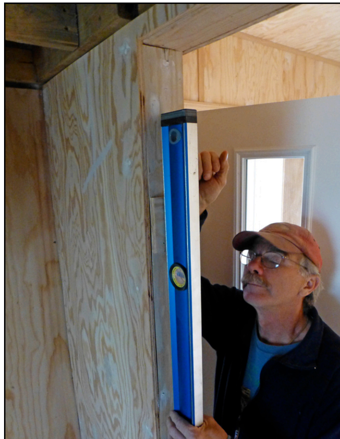
Fig 7.14 Plumbing the hinge side of the door opening with shims prior to door installation.
