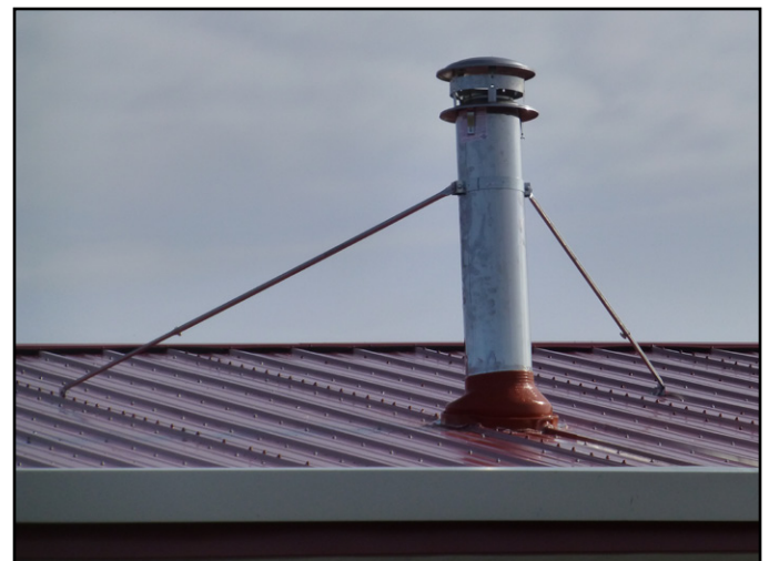
Fig 8.13 The stack for the woodstove should be sealed with flexible boot or a thin-gauged metal chimney flashing and silicone. The stack should be a minimum of 2 feet higher than the ridge if located less than 10 feet from the ridge.
