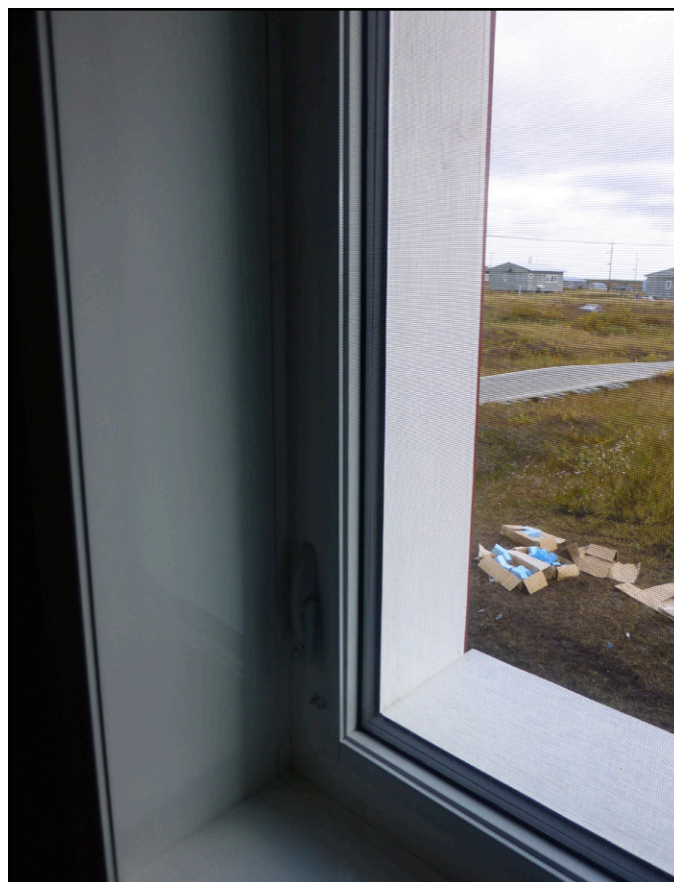
Figure 9.8 The interior window trim consists of an integrated PVC return. The trim should be measured in the field before the windows are placed to depth.
