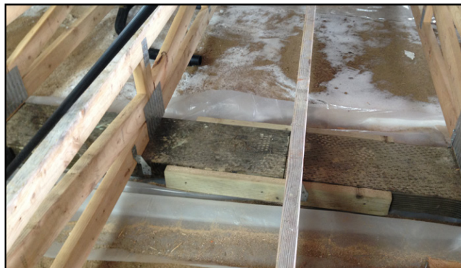
Figure 1.4 In Buckland, the Integrated Trusses are mechanically fastened to treated grade beams on a built-up gravel pad.
