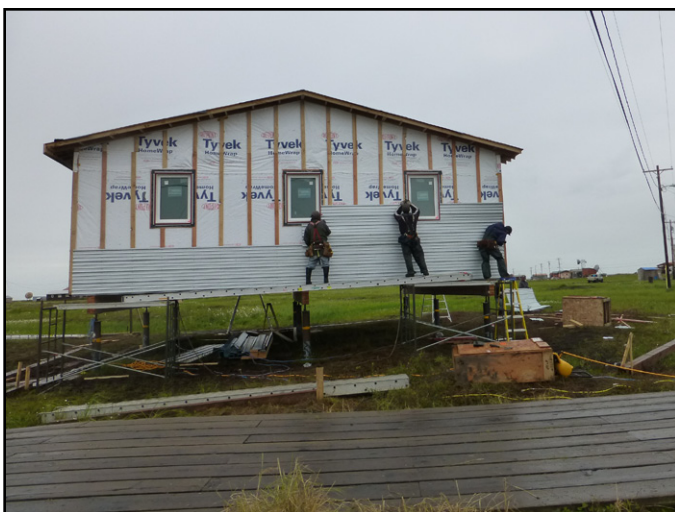
Fig 4.12 Installing siding. The siding is oriented horizontally for less cuts and to allow lateral ventilation of the rain screen. The upper course overlaps the lower.
