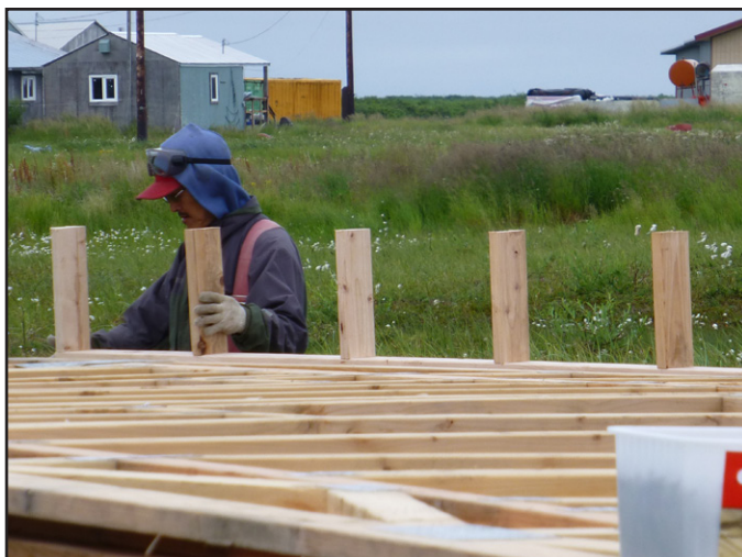
Fig 3.12 If prefabricated spacers are unavailable, they may be made with dimensional lumber on site. 2x blocks pre-installed on each truss to assure proper spacing (12"OC or 24"OC). PRE-INSTALL ALL BLOCKING BEFORE RAISING THE TRUSS.
