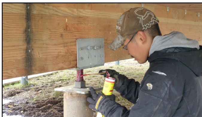
Figure 1.3 Glu-lam beams in Atmautluak are connected to steel piles via an adjustable saddle bracket. The bracket allows for the occupant to re-level the home should any changes in the permafrost create movement in the foundation.
