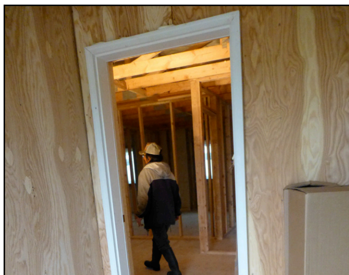
Fig 7.15 Door frame installed.
