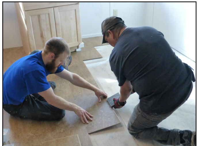
Figure 9.4 Click-in-place flooring is placed directly on top of the tongue-in-groove subfloor. The joints are staggered for added cohesion.
