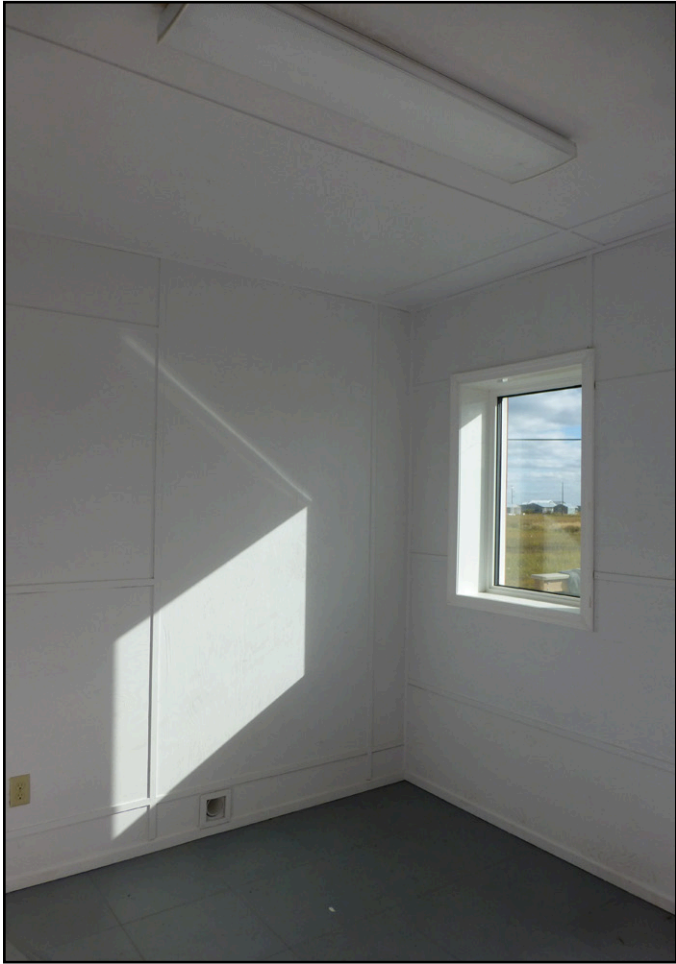
Fig 9.1 Batten strips have been placed before painting.
