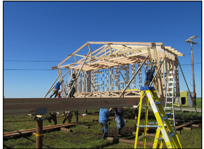
Figure 0.6 Trusses are tipped-up without heavy equipment by an all-local crew and one CCHRC Instructor in the Yukon/Kuskokwim Delta village of Atmautluak.
