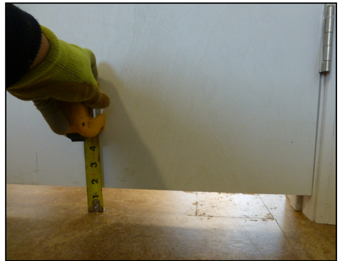
Fig 8.11 The doors of the bedrooms are undercut to leave a 1-1/2" minimum air space. This will allow stale air to return to the HRV and maintain an even temperature throughout the house.
