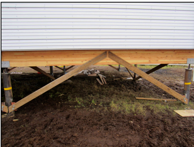
Fig. 2.7 Depending on the height of the foundation, lateral bracing may be required. This bracing is assembled with mechanical connections to a welded tab on the steel piles and to the glu-lam beams. In adjustable foundations, bracing will need to be unconnected during future re-leveling of the home.
