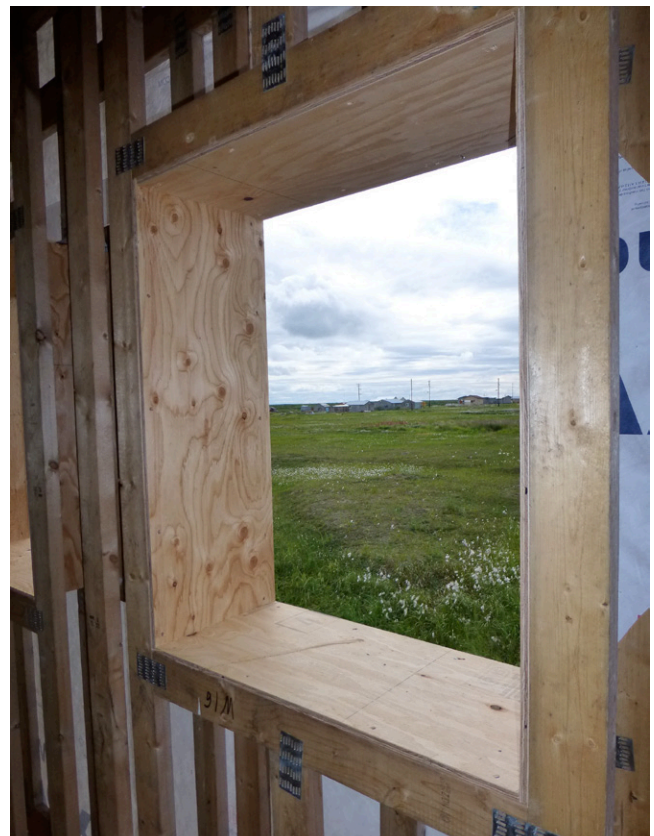
Fig 4.8 The sheathing for the window jamb is installed after the rain screen is completed.
