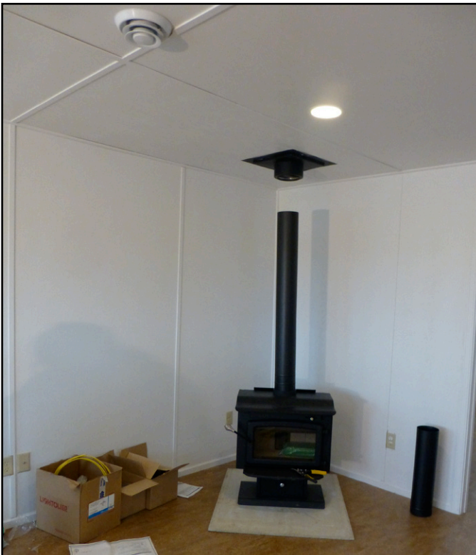
Fig 8.12 The woodstove sits atop a fiber cement board platform. This model of woodstove has integrated heat shields, so that fiber cement board is not necessary on the walls behind the stove. Woodstoves without heat shields will need thermal protection from walls that complies with local fire codes. This stove comes with a direct-vent kit to limit backdrafting.
