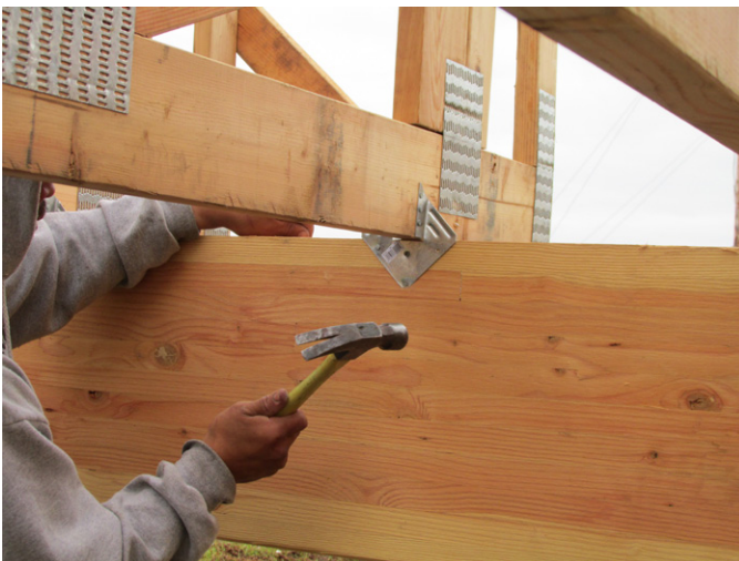
Fig 2.12 Hold-Down connection for the glu-lam beam scenario.
