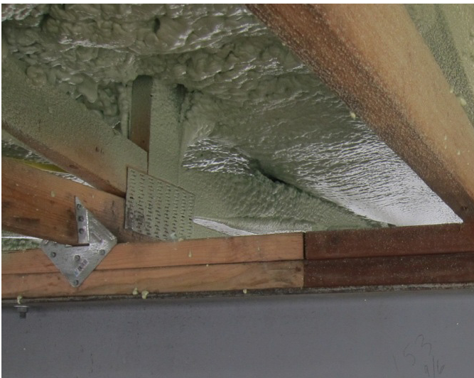
Fig 2.10 Hold-Down connection for the steel beam scenario requires double sill plates.
