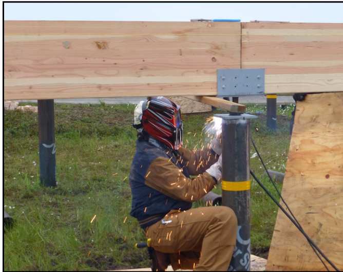
Fig 2.5 Once the beams are square and level, the bottom plate of the bracket assembly is welded to the top of the steel pile.
