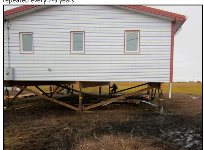
Fig 2.8 If lateral bracing is required, it should be applied along both axes of the home.
