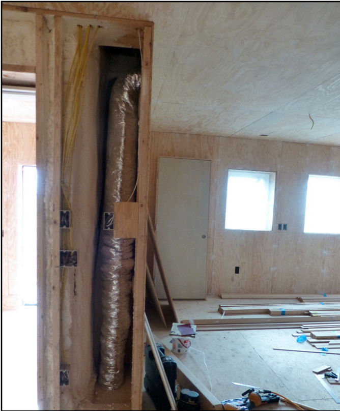
Fig 8.9 A 6" passive makeup-air vent is installed behind the refrigerator to provide supply air when exhaust appliances such as the kitchen fan is turned on. The ducting from the floor intake to the room must be insulated.
