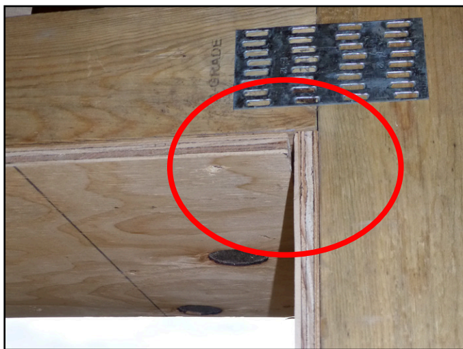
Fig 5.1 Plywood window jambs installed. Note plywood at top and bottom installed after sides to prevent closed cell insulation from distorting jambs.
