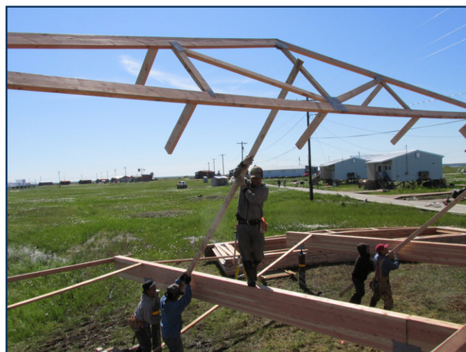
Fig 3.13 Erecting trusses using 2x4 push poles.
