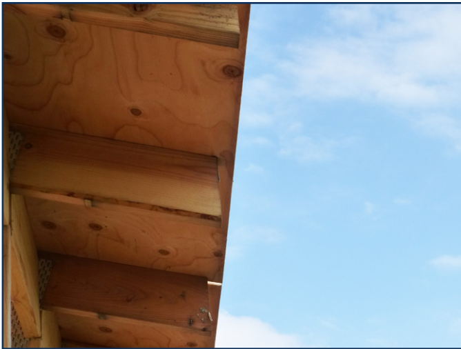
Fig 4.6 Plywood sheathing extends 1 1/2" beyond top chord of roof truss. It will cover top edge of 2x sub-facia.
