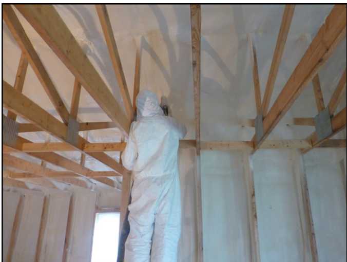
Fig 7.1 Installing closed cell foam. The roof and walls are sprayed in one continuous coat to form a monolithic thermal envelope. The foam is applied in 2" lifts.
