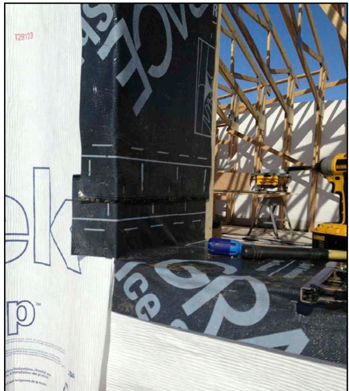
Fig 5.7 Ice and water shield wrap around window rough opening. This photo is not from the Pikat Construction job.
