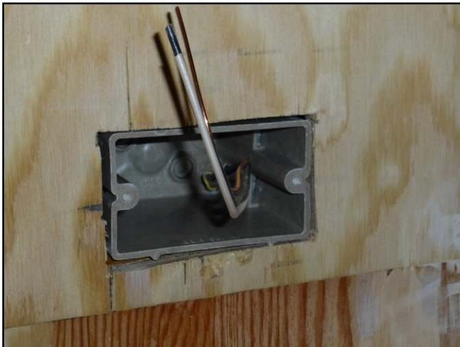
Fig 9.3 Electrical rough-in box. When using AC Plywood interior finishes instead of gypsum wall board, oversize plate covers should be ordered.
