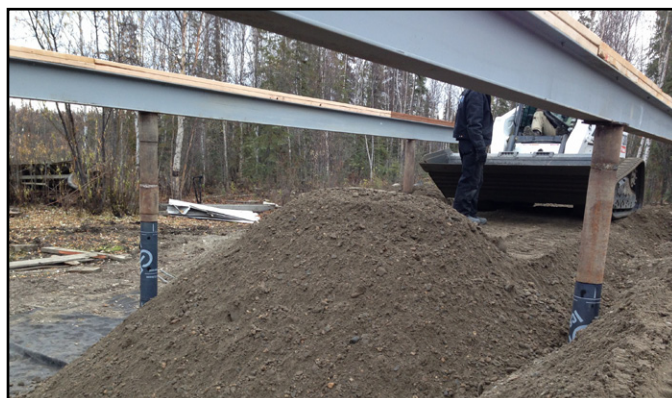
Figure 1.2 Steel piles welded to steel wide flange beams keep a replacement home above the 100-year floodplain in Galena. The Integrated Trusses will be erected atop the wood double top plate.
