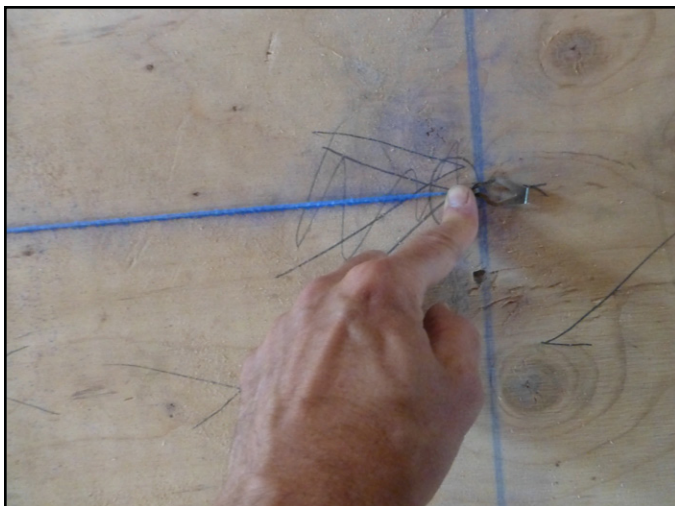
Fig 7.6 Lay out interior walls with chalk line.
