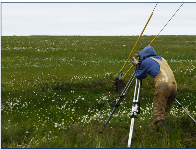
Fig 2.1 Using a builder's level, the base of each crib/pile/etc is brought to the same elevation.
