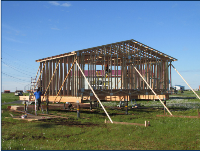
Fig 3.16 Trusses \frac{3}{4} installed. Note diagonal bracing with 2x4s. In this early version, shear panels were not required in this region. Check the plans for shear panel blocking requirements.
