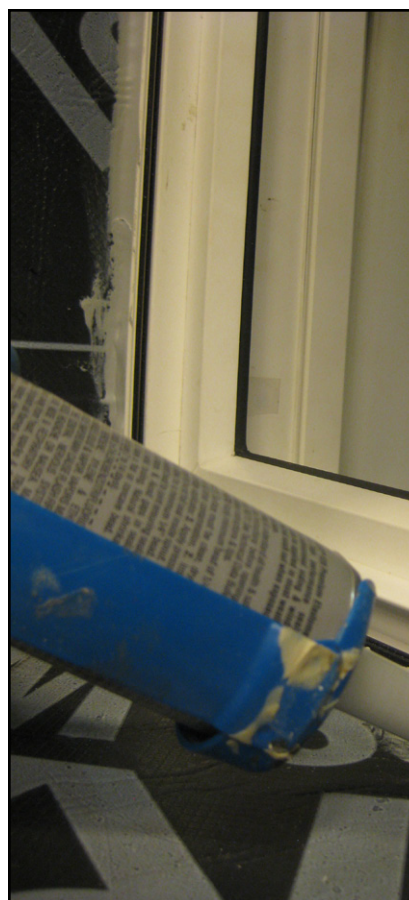
Fig 5.9 Installing caulking at gap between window and framing at exterior face
