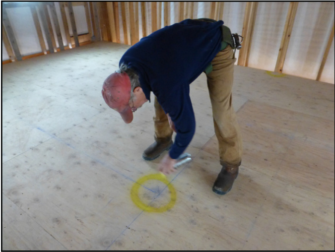
Fig 7.8 Corners are marked for interior layout.
