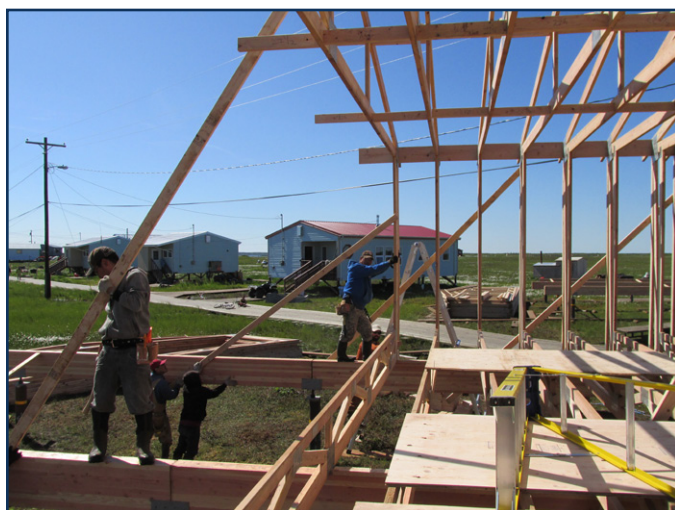
Fig 3.14 Trusses installed. Note: Plumbing each truss is not necessary if first truss is installed correctly.
