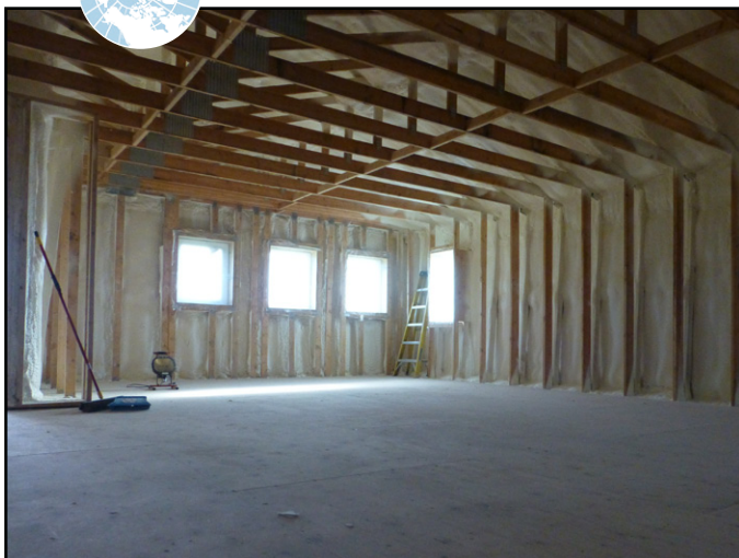
Fig 7.3 View of installed closed cell foam.
