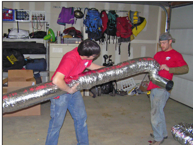
Fig 8.5 Ducting to the outside must be insulated. Insulated flex duct should be avoided, as it will significantly reduce airflow. Instead, 6" smooth wall sheet metal pipe can be insulated by removing the insulation jacket from 7" flex duct and sliding it over the 6" pipes.
