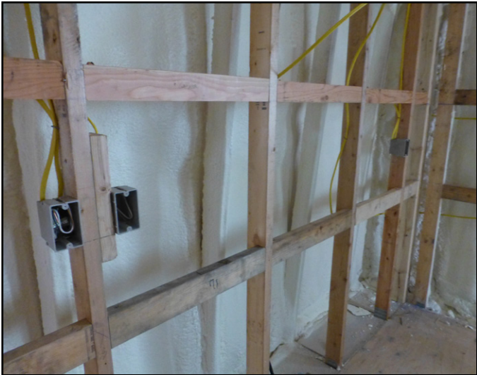
Fig 7.10 Blocking installed for kitchen cabinets and duplex outlet.
