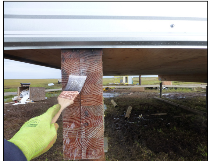
Fig 2.6 The cut ends of the beams are treated with a water seal coating. The long edges of the windward sides of the beams may also be water sealed to ensure the glu-lam's longevity. This should be repeated every 2-3 years.
