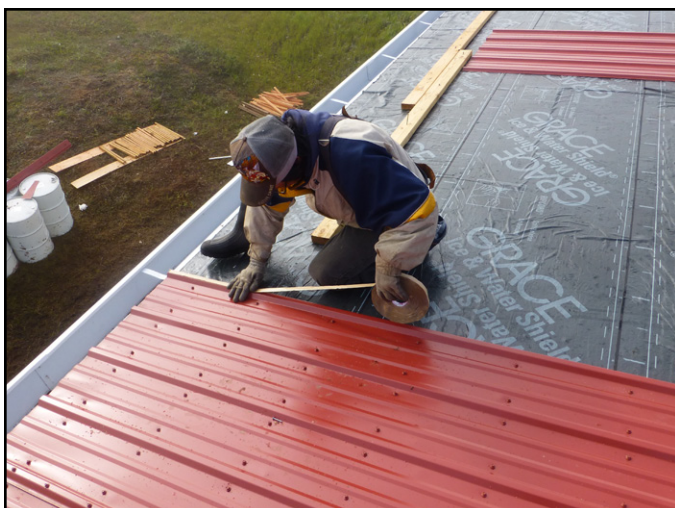
Fig 6.3 Metal roof installation. It is important to comply with the fastener schedule provided by the metal roof manufacturer. Note 2-sided tape at roof panel overlap.
