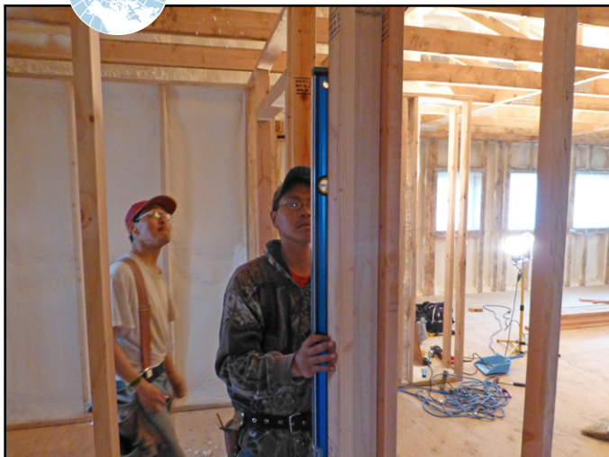
Fig 7.13 Plumbing the hinge side of the door opening with shims prior to door installation.
