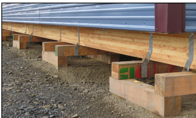
Figure 1.1 The Integrated Truss home in Crooked Creek rests on Glu-lam beams fastened to cribbing with hold-down connections. The cribbing rests on a built-up gravel pad that has been properly compacted.
