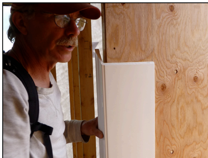
Fig 5.2 Pre-built interior window jamb extensions with casing applied. Determines placement of window in opening and dimensions of site built exterior jamb extensions.
