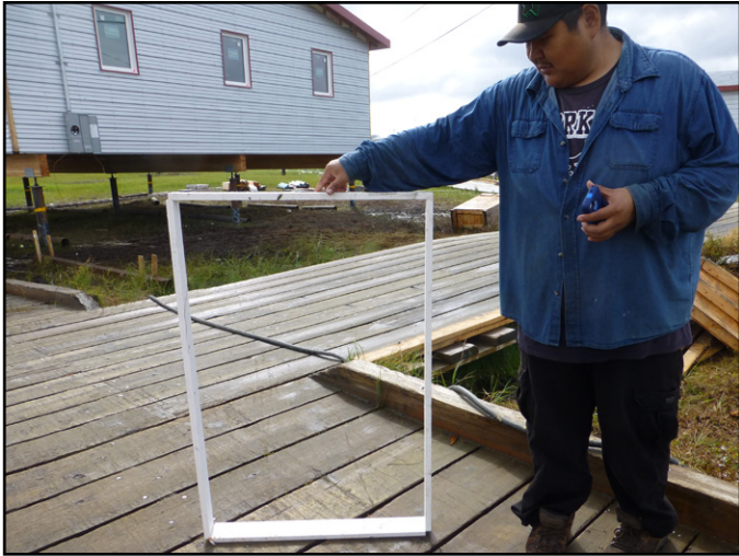
Fig 5.3 Site built exterior window jamb extension.
