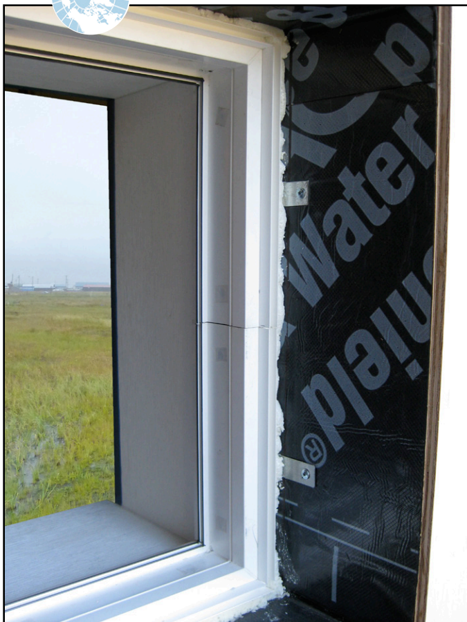
Fig 5.8 Installed windows. The impermeable peel and stick membrane is applied flush with the interior face of the rough opening, and the exterior field-built jam extension is in place. Foam air sealing is in place around the rough opening. The interior prefabricated jamb extension with casing will be attached after painting.
