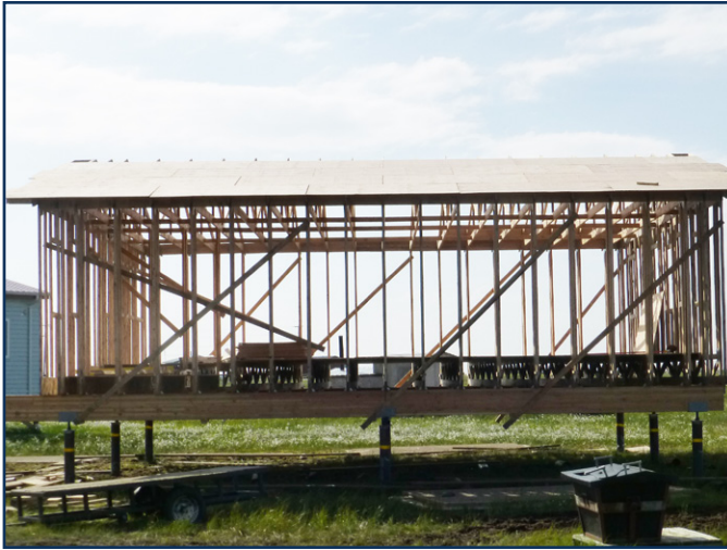
Fig 4.4 Roof sheathing installed on one side of roof. Note plywood for the other side of the roof stacked on the subfloor.
