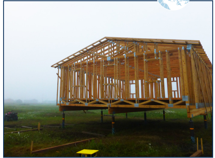
Fig 3.17 Truss and bracing installation complete.
