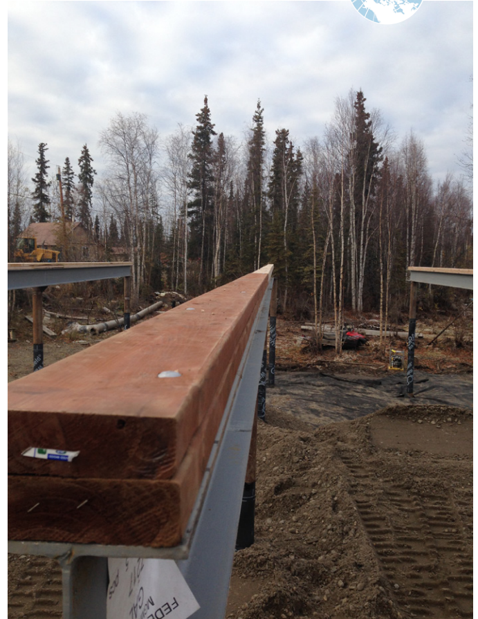
Fig 2.11 Cut sill plates to length and place on top of I-beams.
