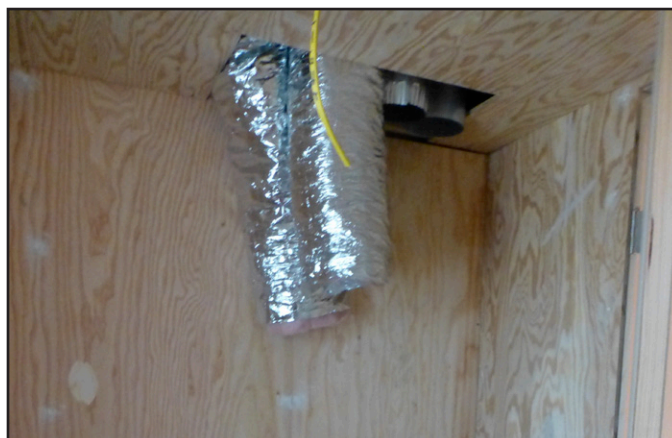
Fig 8.6 Space in the ceiling sheathing must be left so that the HRV can be connected to the ducting. A separate hatch must be left open so that ducting can be installed above the ceiling
