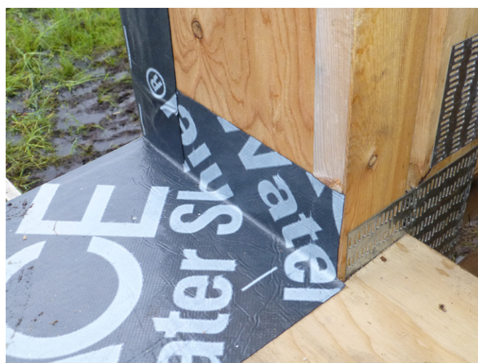
Fig 5.11 Door jamb is detailed with impermeable peel and stick membrane.
