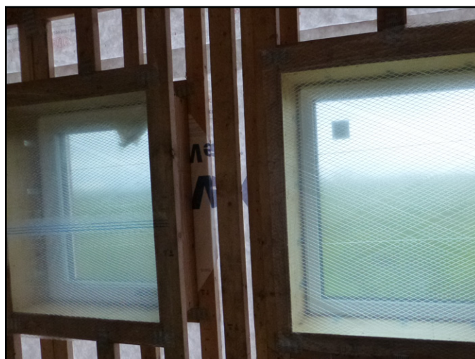
Fig 5.10 Reinforced poly covers windows to prevent over spray from closed cell foam insulation from damaging the windows.
