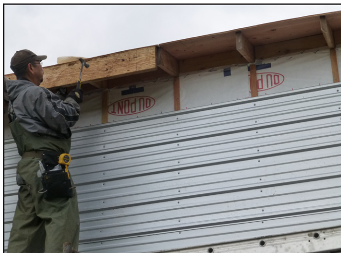
Fig 6.2 Installing 2x sub fascia.
