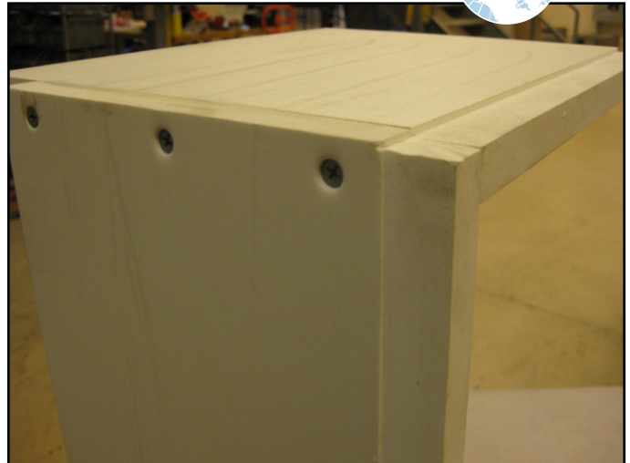
Fig 5.4 Site built window jamb extension rabbeted out to fit into exterior window jamb receiver.
