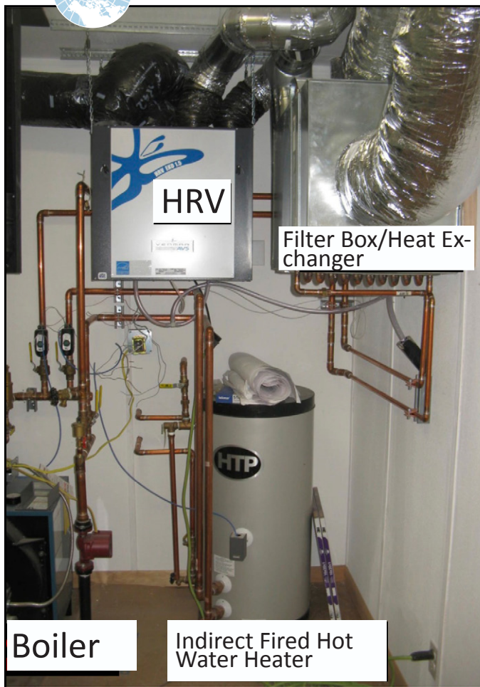
Fig 8.4 View of the mechanical room with a typical BrHEAThe system configuration. HRV unit should be hung from the bottom chord of the truss structure and have a few inches of clearance from surrounding walls to limit vibration. The condensate line must have a trap.
