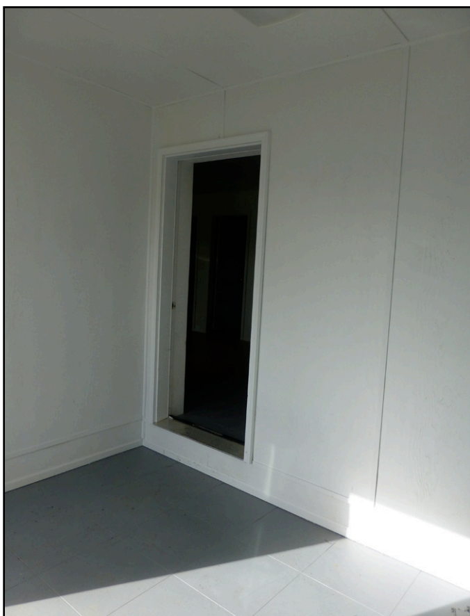
Figure 9.7 The Elaturaq entry door threshold has a PVC extension to accommodate the extra wall thickness. The step up into the home from the entry will help form a passive cold trap.
