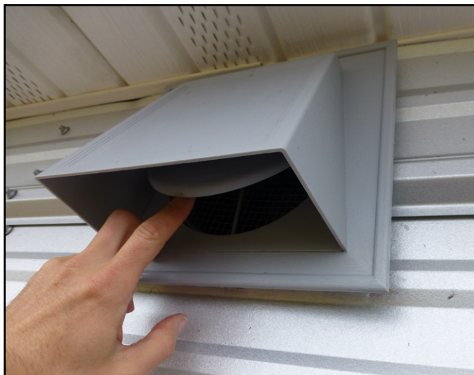
Fig 8.8 The weather hood comes with an integrated hinged flap. The flap should remain in the exhaust hoods, but be removed in the intake hoods.
