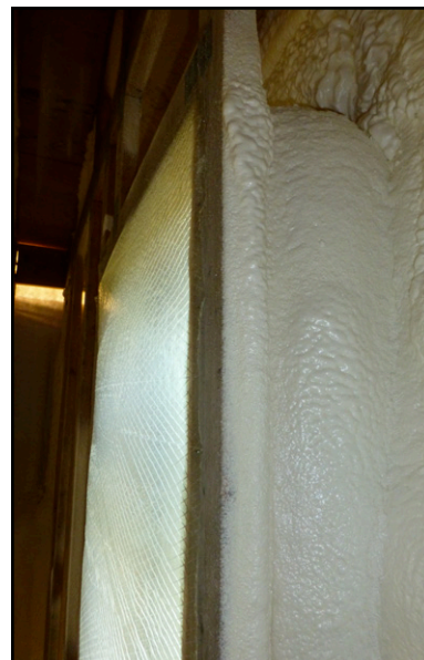
Fig 7.2 Foam installed around plywood window rough opening frame. It is important that the window box have the same thickness of foam as the wall insulation.
