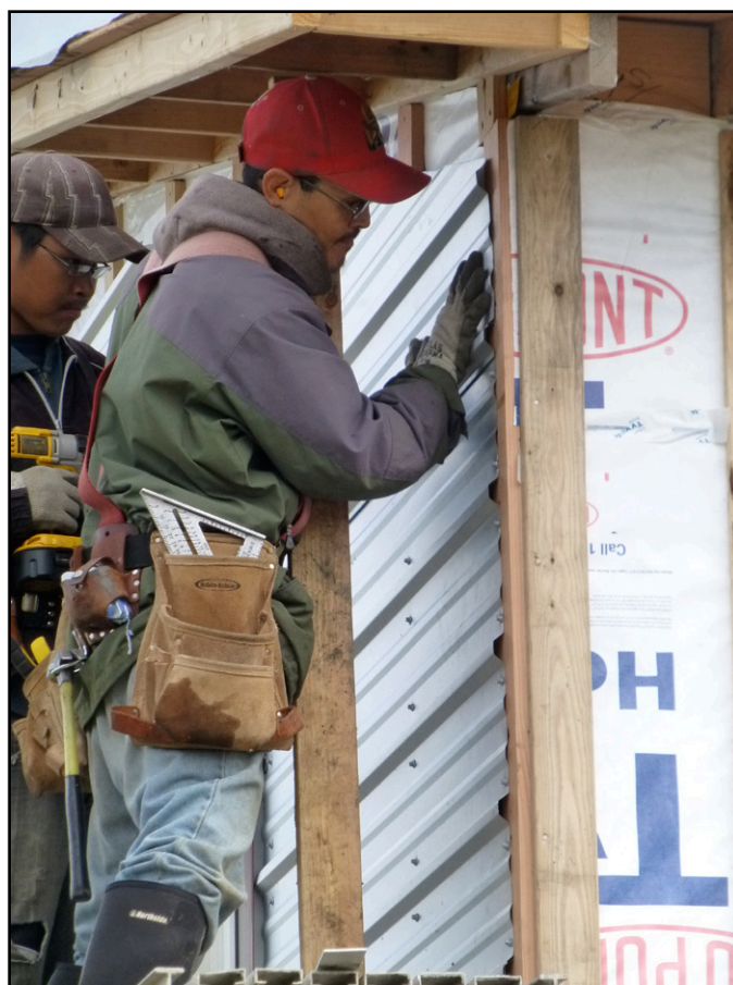
Fig 4.13 Installing siding. Siding is held off the corners and a 90-degree trim will cover the joints.
