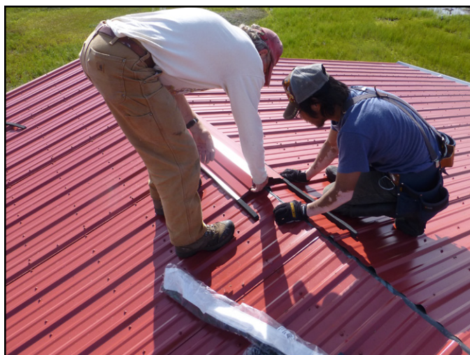
Fig 6.4 Installing metal roof ridge cap and inside closure pieces to keep rain from getting under the cap.
