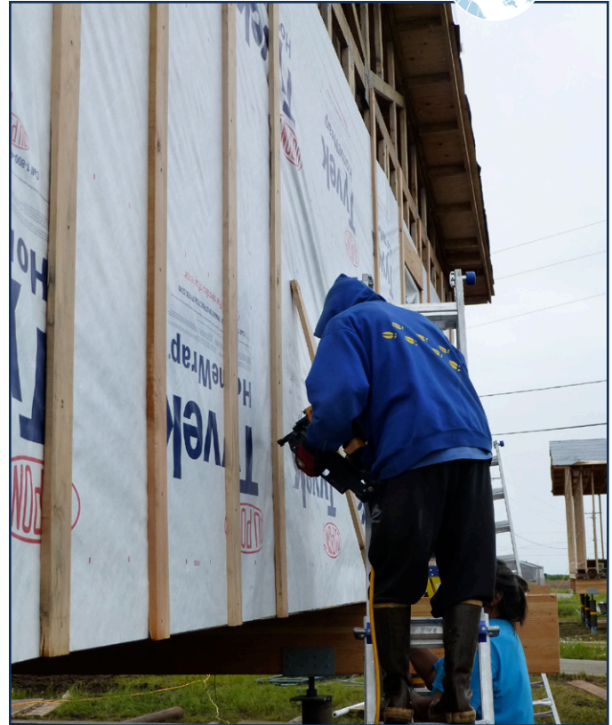
Fig 4.5 Installing 1x spacers for rain screen.
