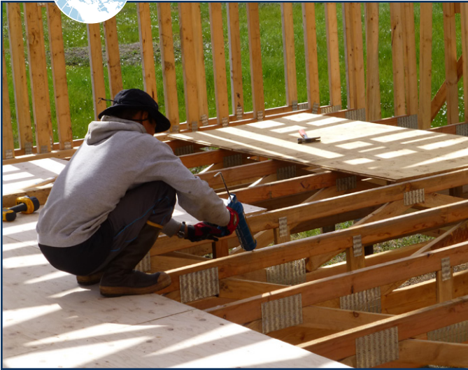
Fig 4.2 Applying construction adhesive to the top chord of each floor truss prior to the installation of the plywood subfloor. In this scenario, the insulation will be sprayed upwards from below.
