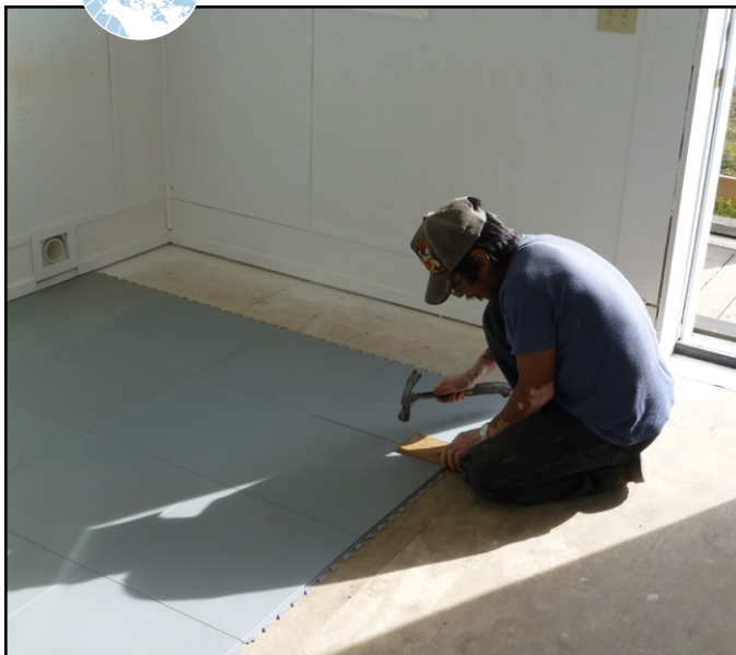
Figure 9.5 The rubber floor tiles can be connected using a rubber mallet or a hammer and block.
