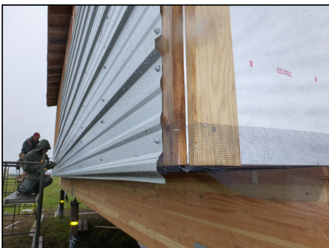
Fig 4.11 Installed metal siding. Note siding is held 1" below bottom chord to hide edge of 3/8" plywood that will form the underside sheathing after the floor is insulated from below.
