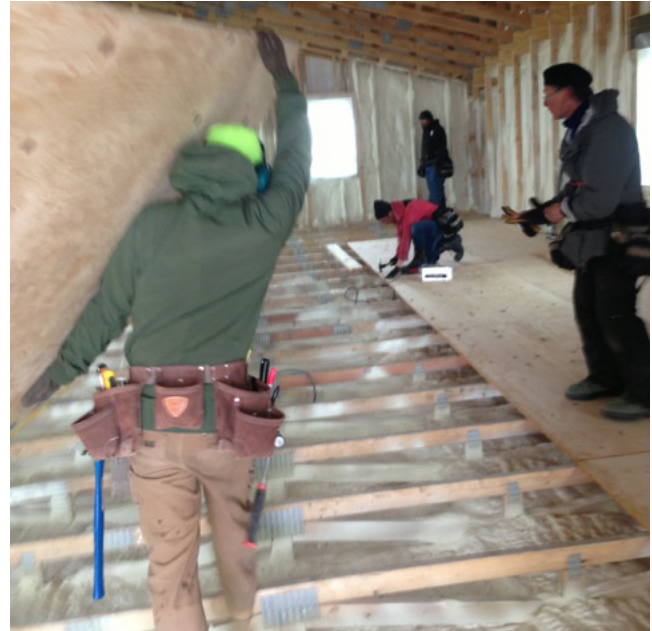
Fig 4.3 In this scenario, insulation was sprayed from above. Subfloor is fastened permanently in place after spraying is complete.
