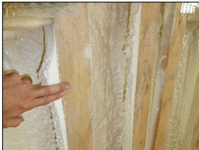
Fig 7.4 Foam at exterior wall intersection. After application, the excess foam must be removed from the studs so interior sheathing is uniform and flush.
