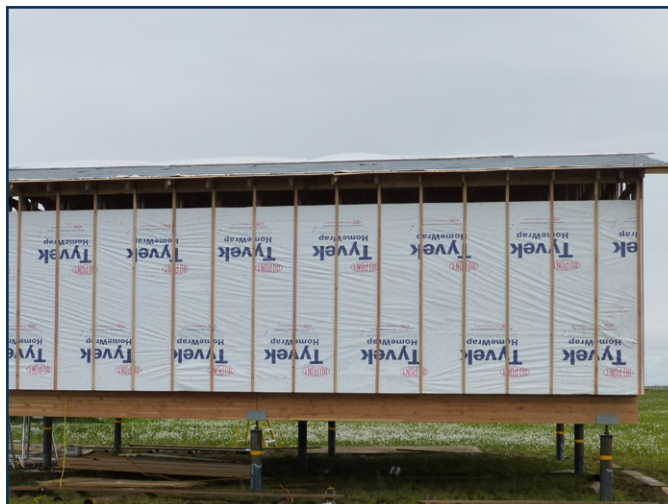
Fig 4.7 Tyvek rain screen and 1x spacer blocks installed over the exterior chord of the wall truss.
