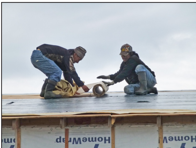
Fig 6.1 Installing ice and water shield over plywood roof sheathing.
