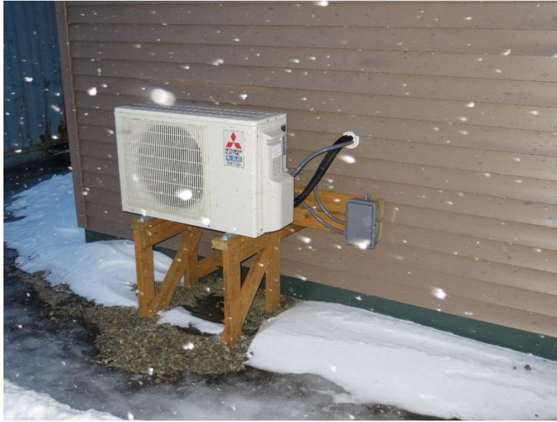
Figure 5. Outdoor unit of the Mitsubishi heat pump in Dillingham.
