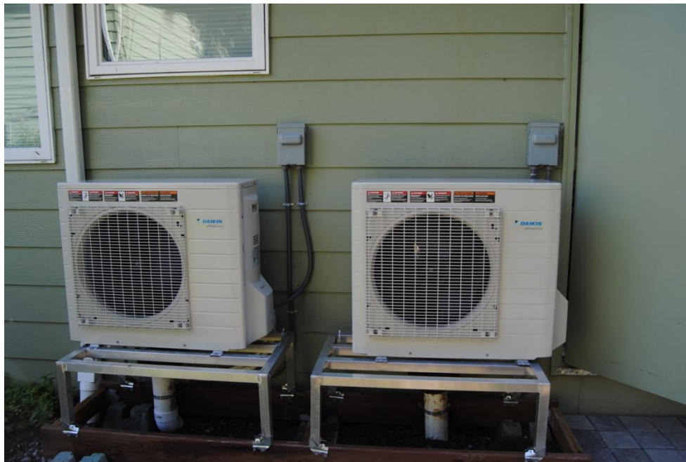
Figure 7: The outdoor units for the Juneau heat pump.
