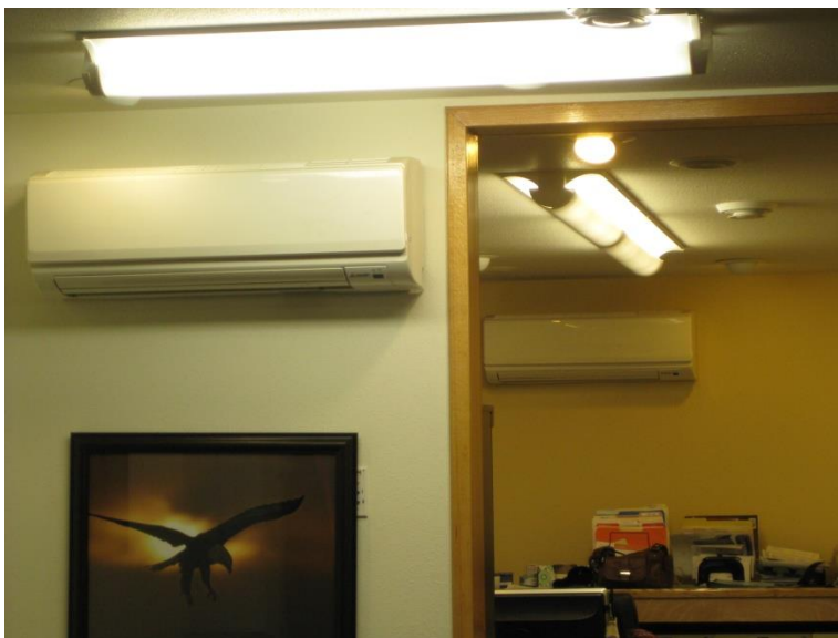
Figure 2: Two indoor units for a ductless heat pump system.
