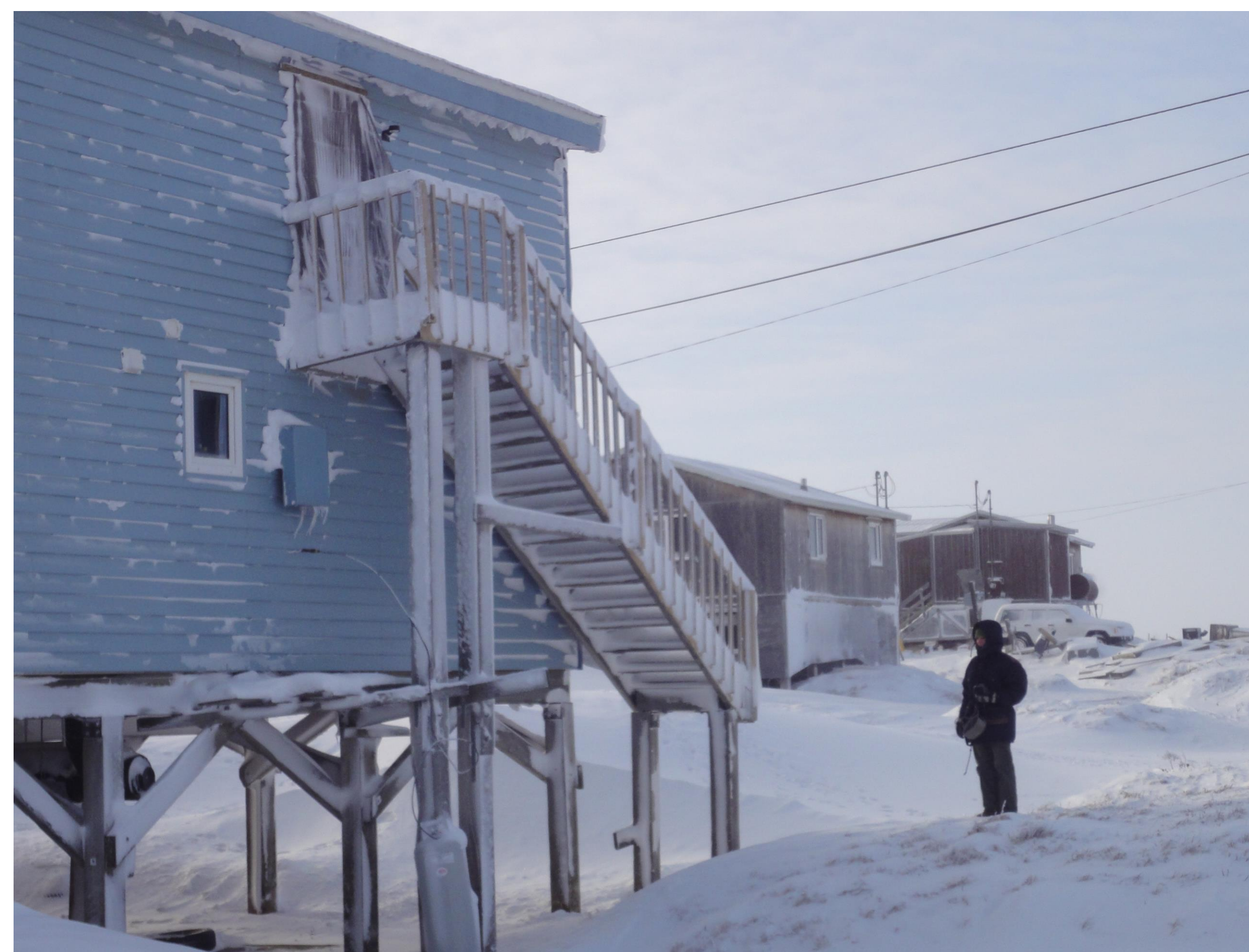
A building in Point Lay, AK that has been affected by permafrost thaw. Ground subsidence has left the stairs nearly seven feet off the ground, but because the piles have been driven so deep into the permafrost layer that the building is level and intact.
