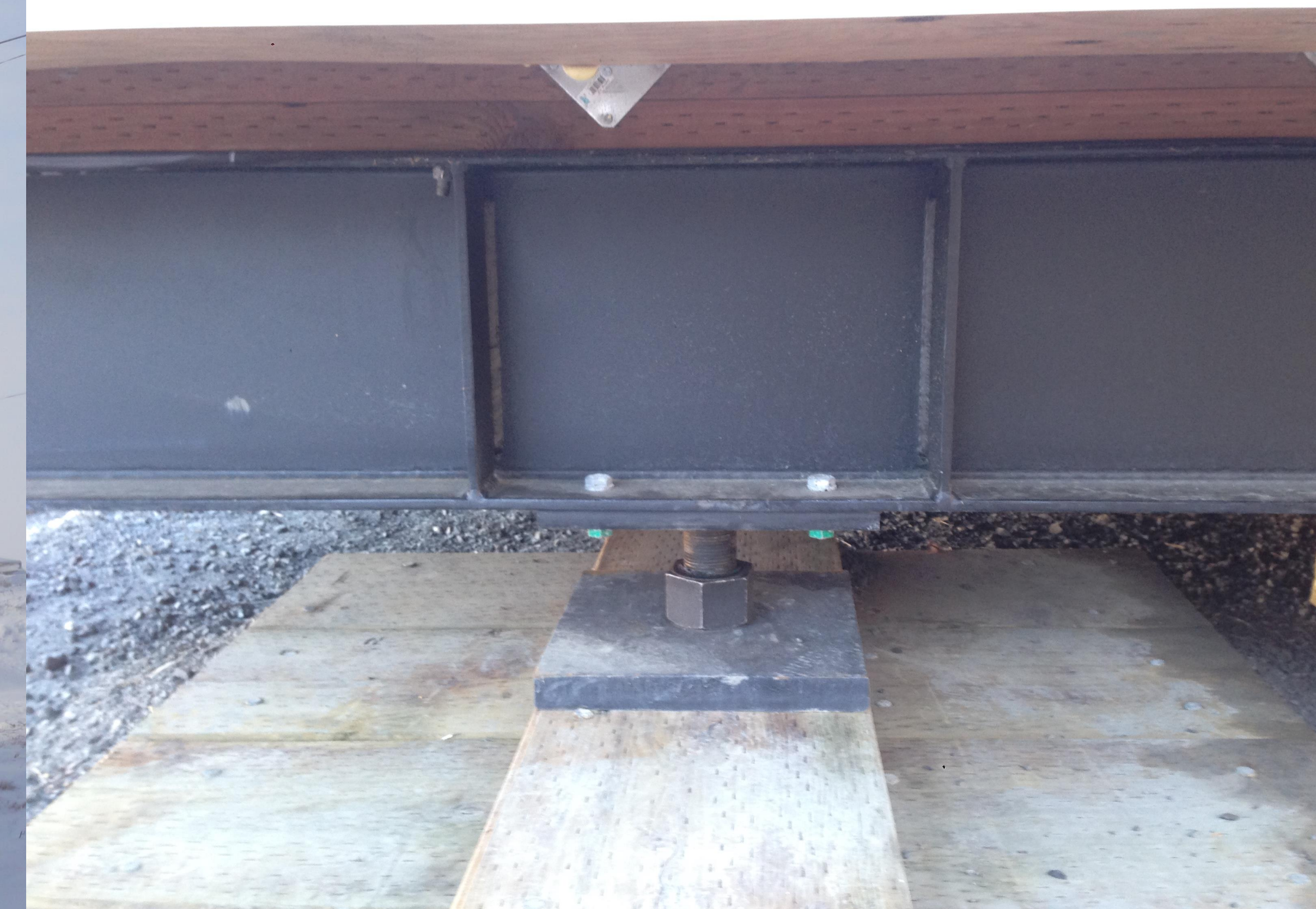
An example of a post and treated wood pad foundation.
