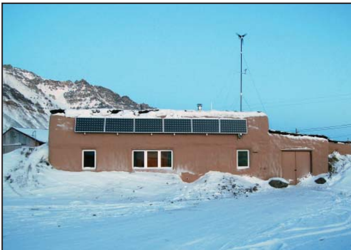
Completed prototype home with solar photovoltaic and wind power installations
