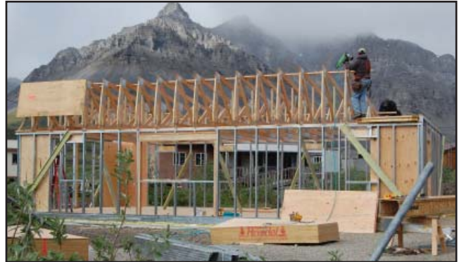
Prototype house in construction June 2009
