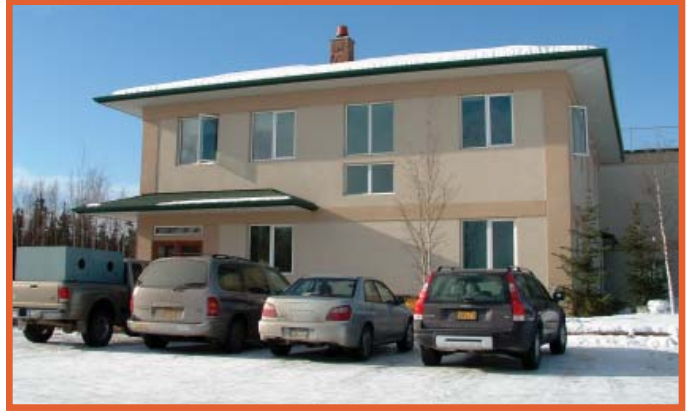
The Cold Climate Housing Research Center Research and Test Facility in Fairbanks, Alaska.
