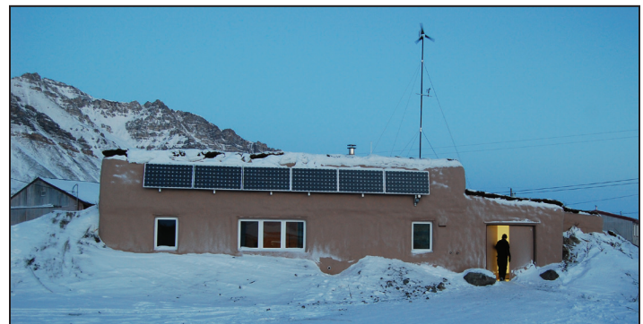
The prototype home in AKP has a highly insulated thermal envelope to minimize fuel demand.
